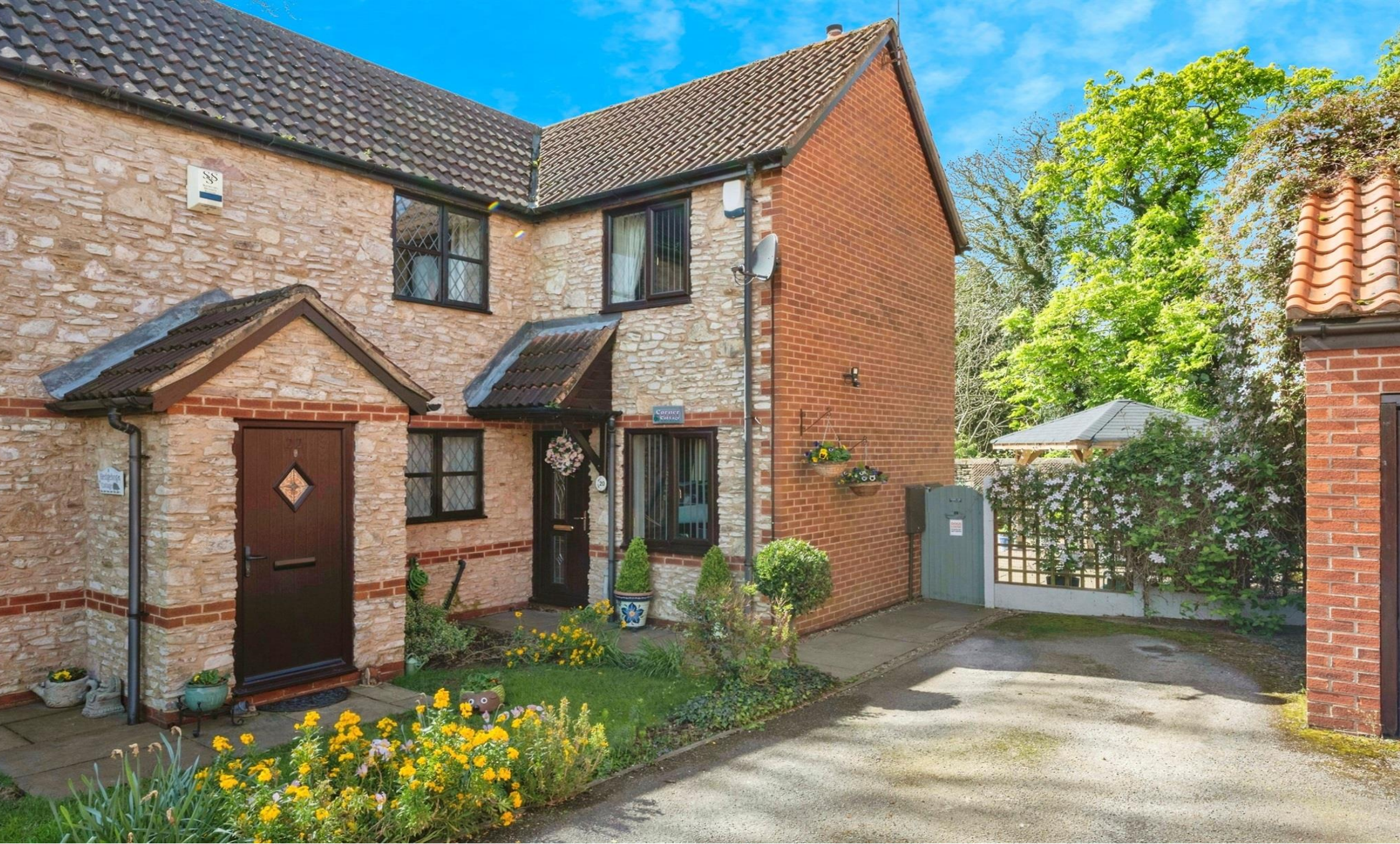
South Farm Drive, Skellow Doncaster
