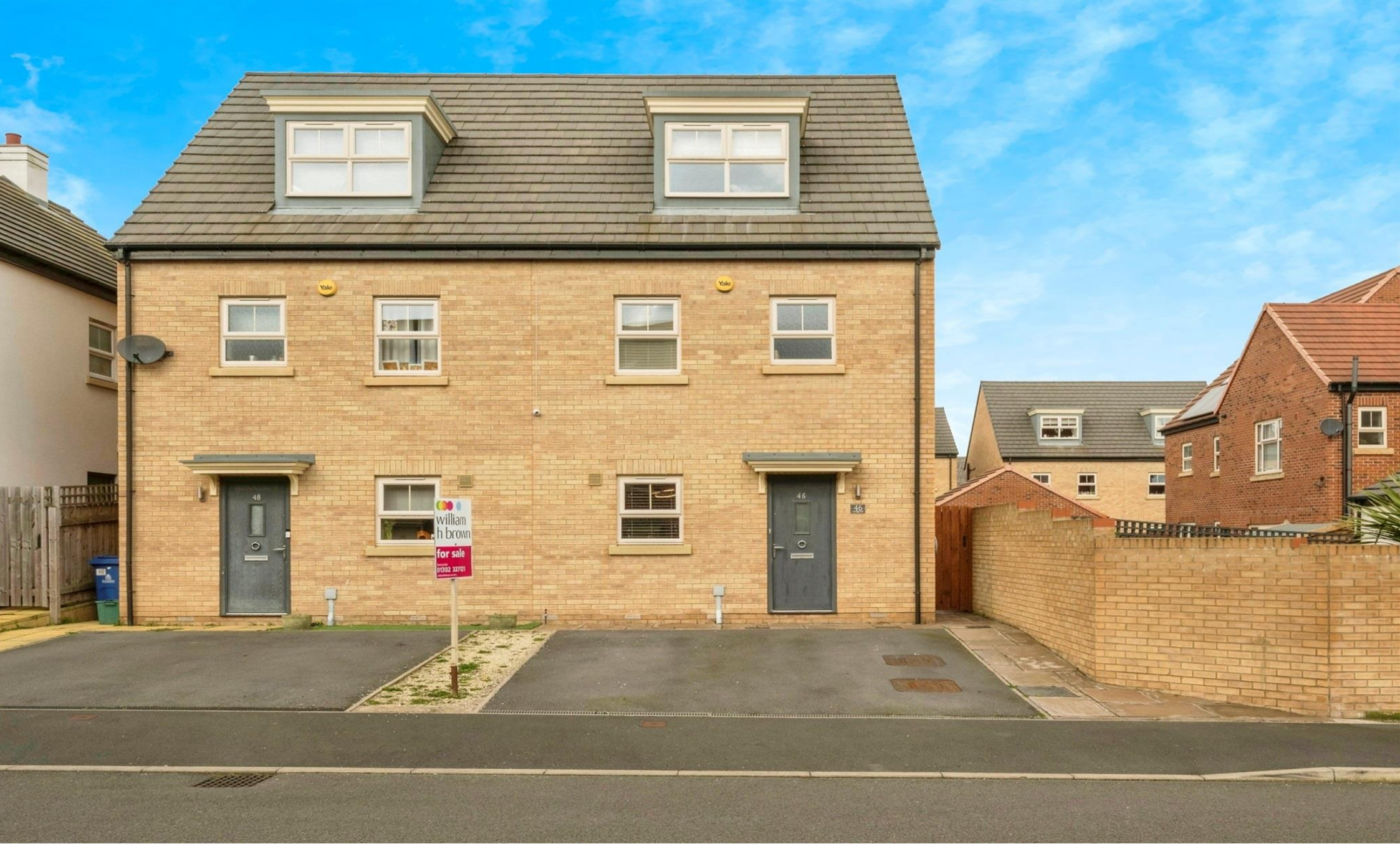
Stretton Street, Adwick-Le-Street Doncaster
