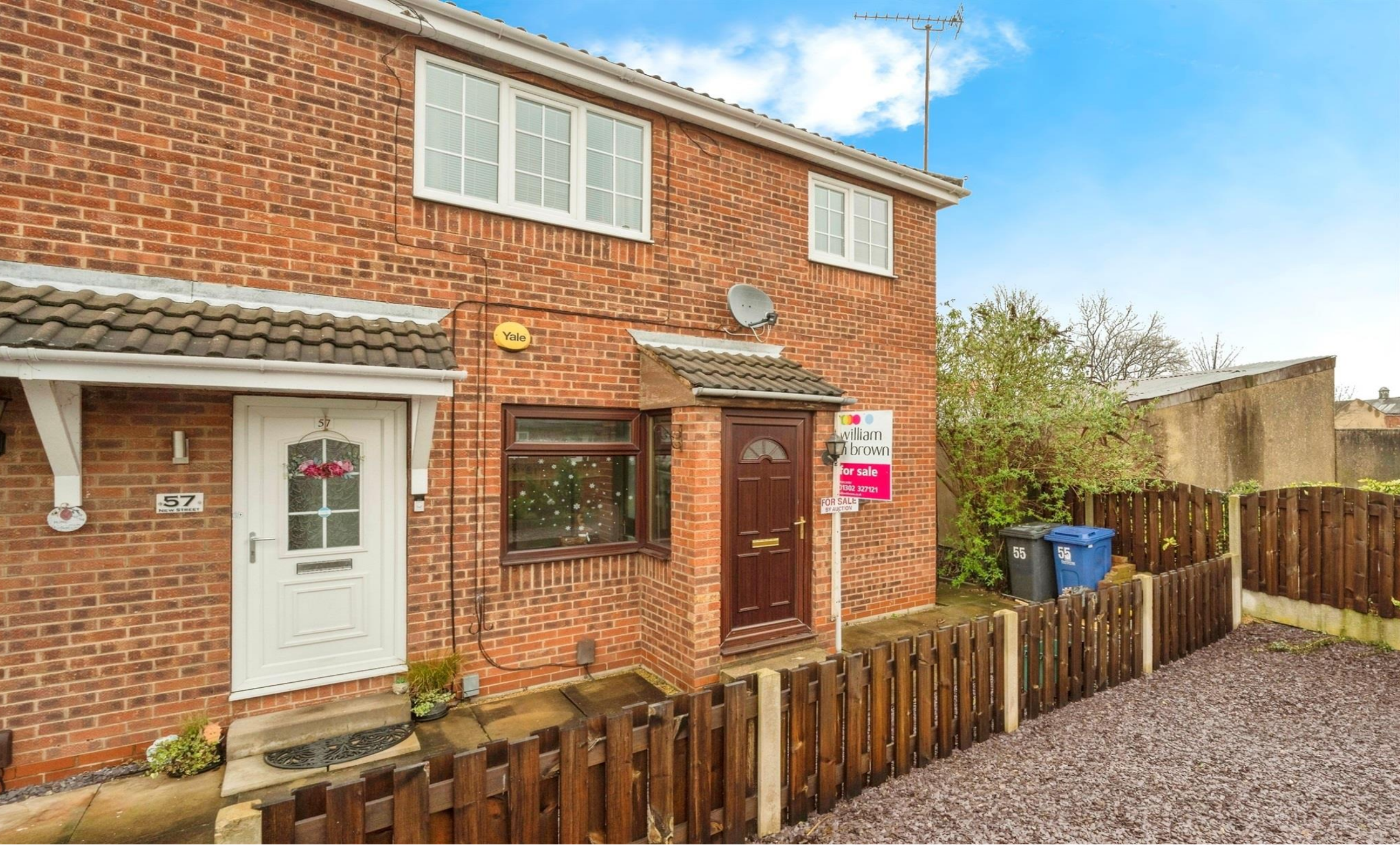
New Street, Bentley Doncaster
