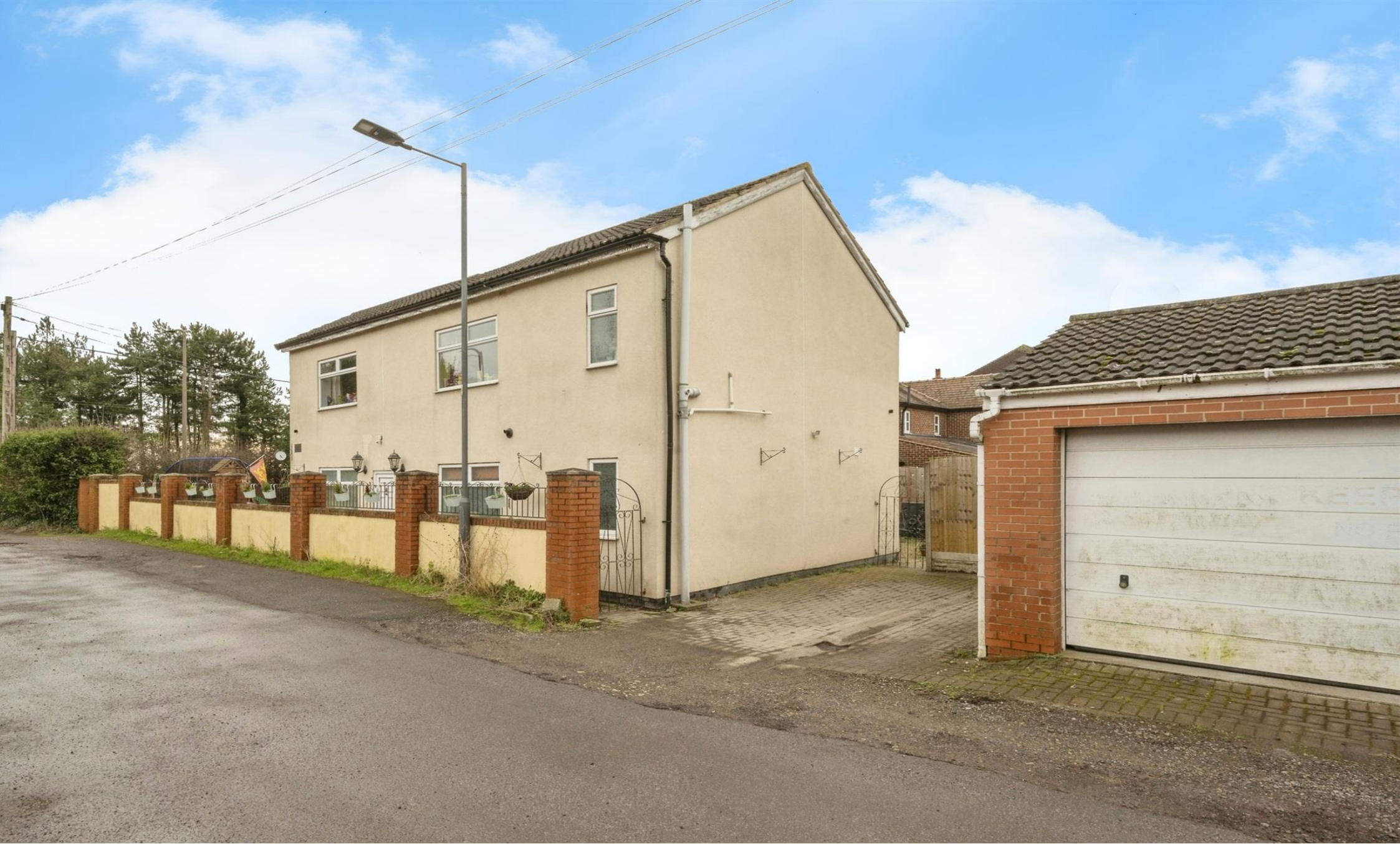
Douglas House Station Road, Blaxton Doncaster
