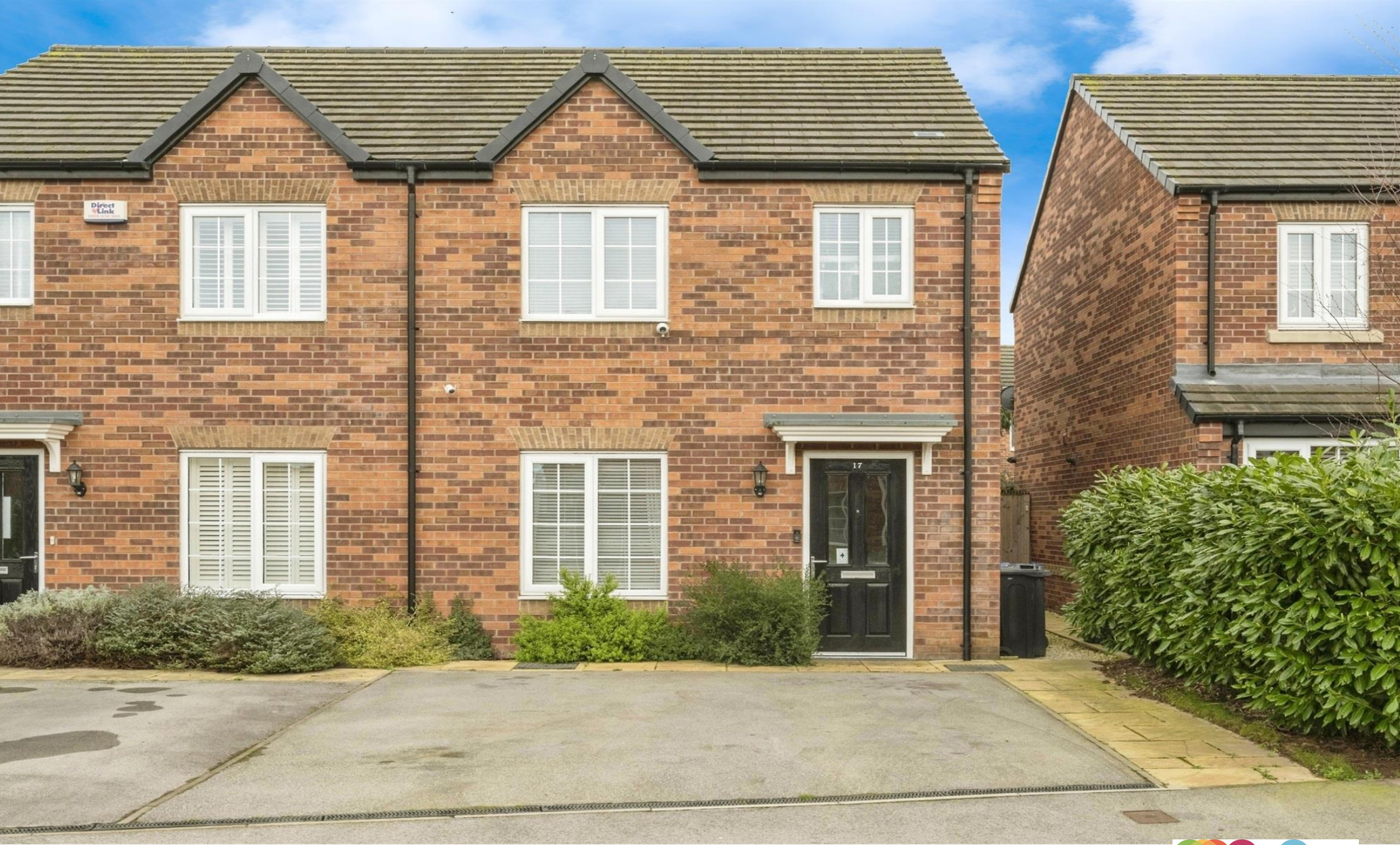
Heatherfields Crescent, New Rossington Doncaster
