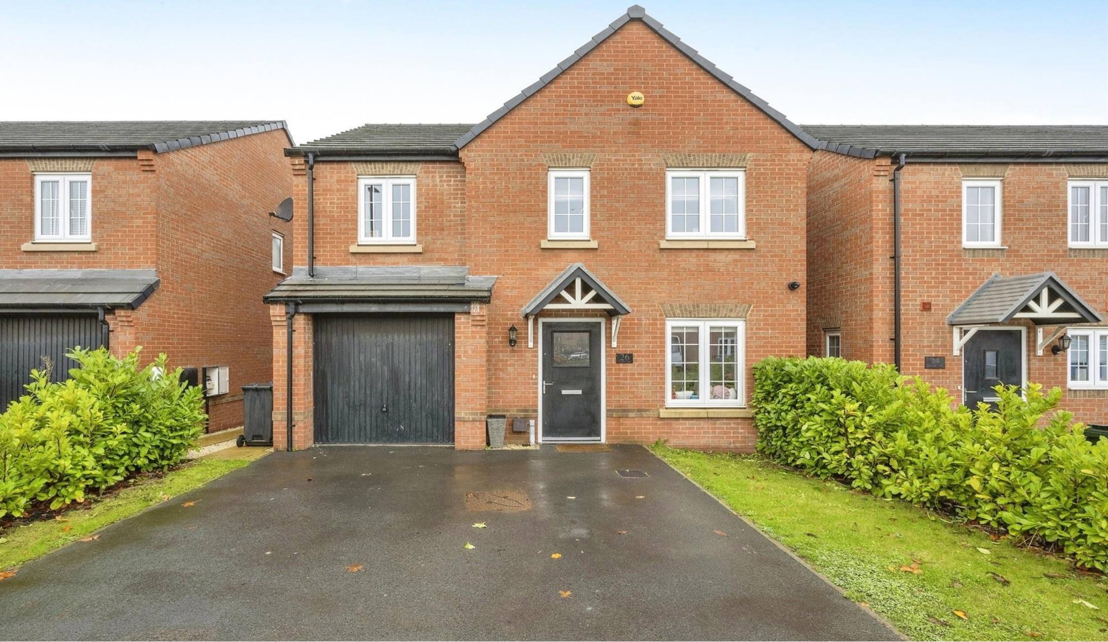
Cutter Lane, New Rossington DONCASTER
