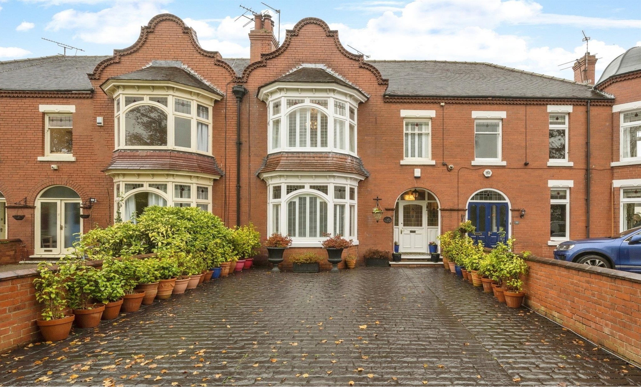
Town Moor Avenue, Town Moor Doncaster
