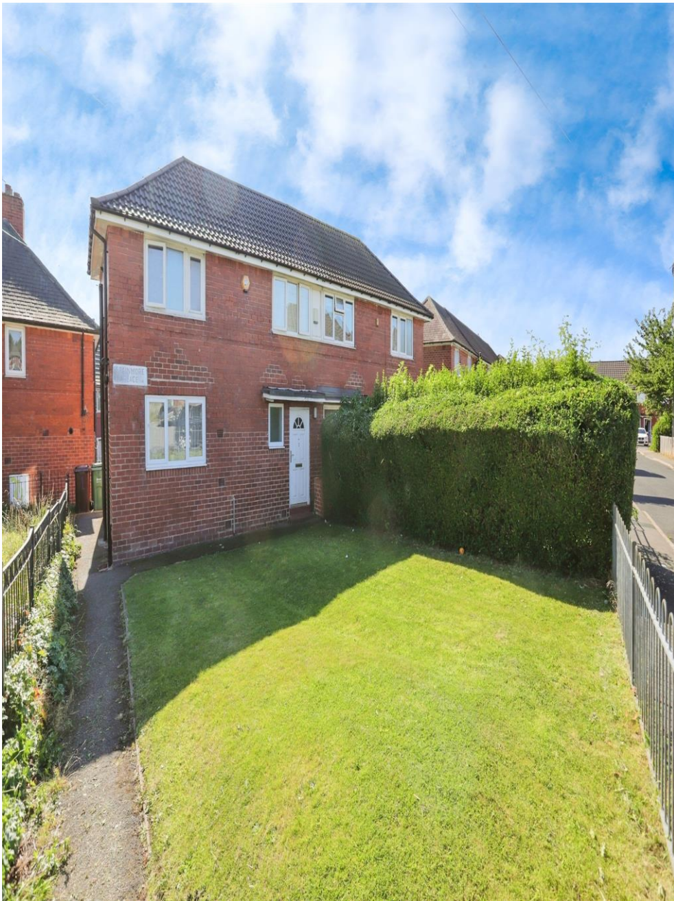
Stainmore Place, Leeds LS14 6BU
