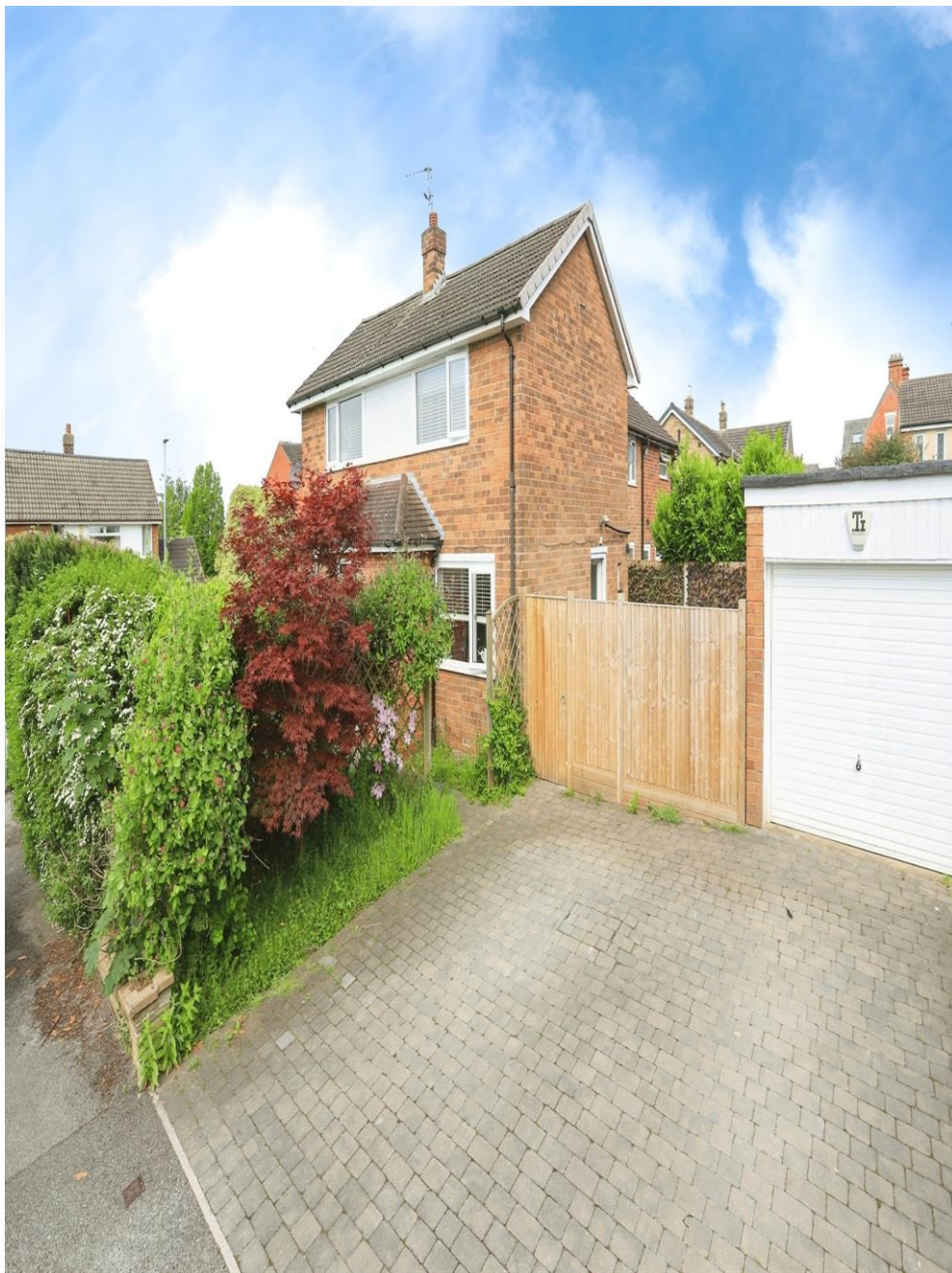
Rectory Close, Garforth Leeds LS25 1HH
