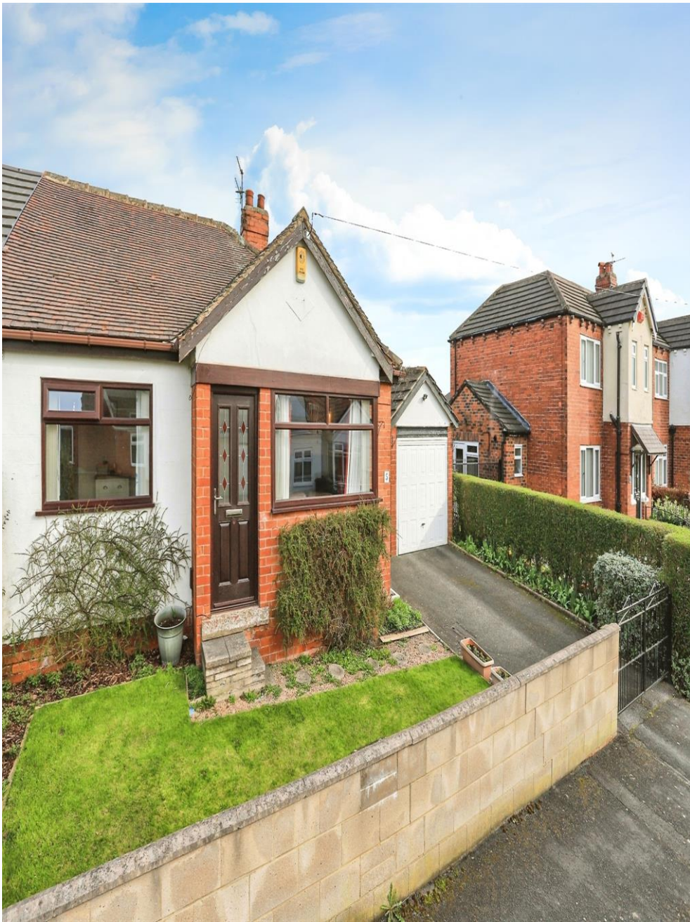
Howard Avenue, Leeds LS15 0LZ
