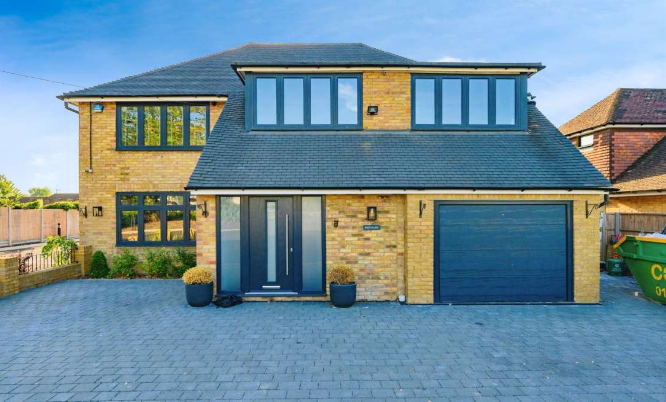
Mehalah High Street Green, Hemel Hempstead HP2 7AQ
