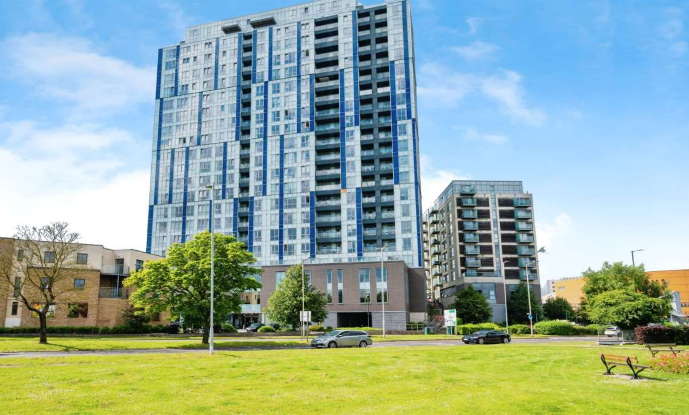
Kd Tower Cotterells, Hemel Hempstead HP1 1AT
