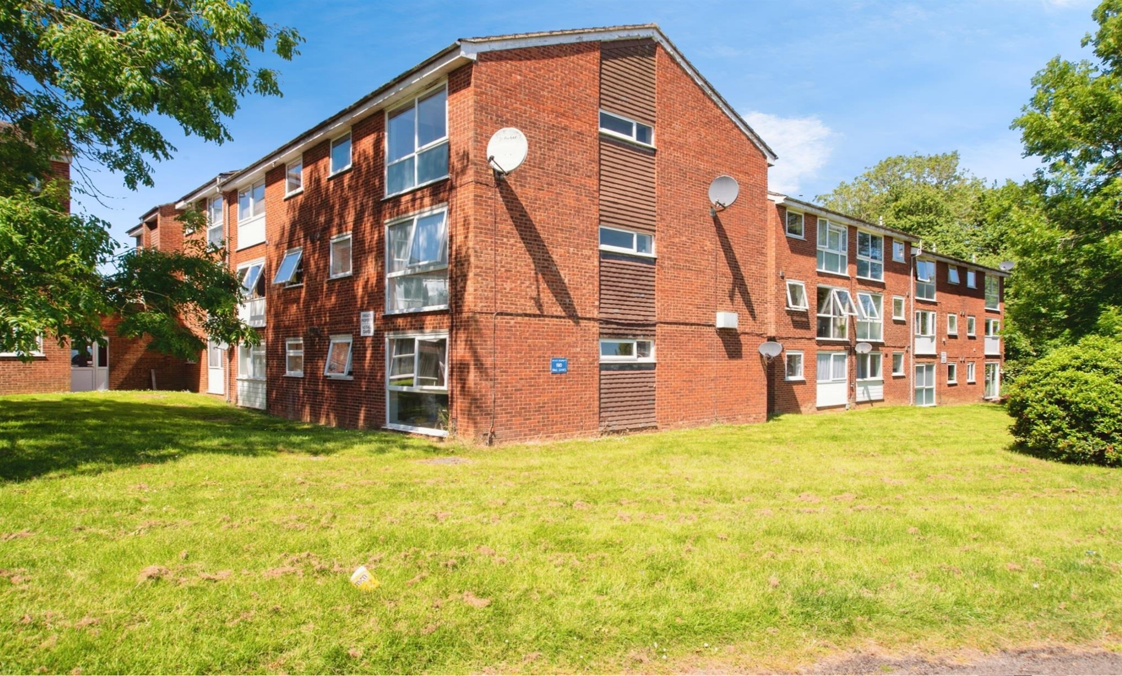
Roydon Court, Hemel Hempstead HP2 7PA
