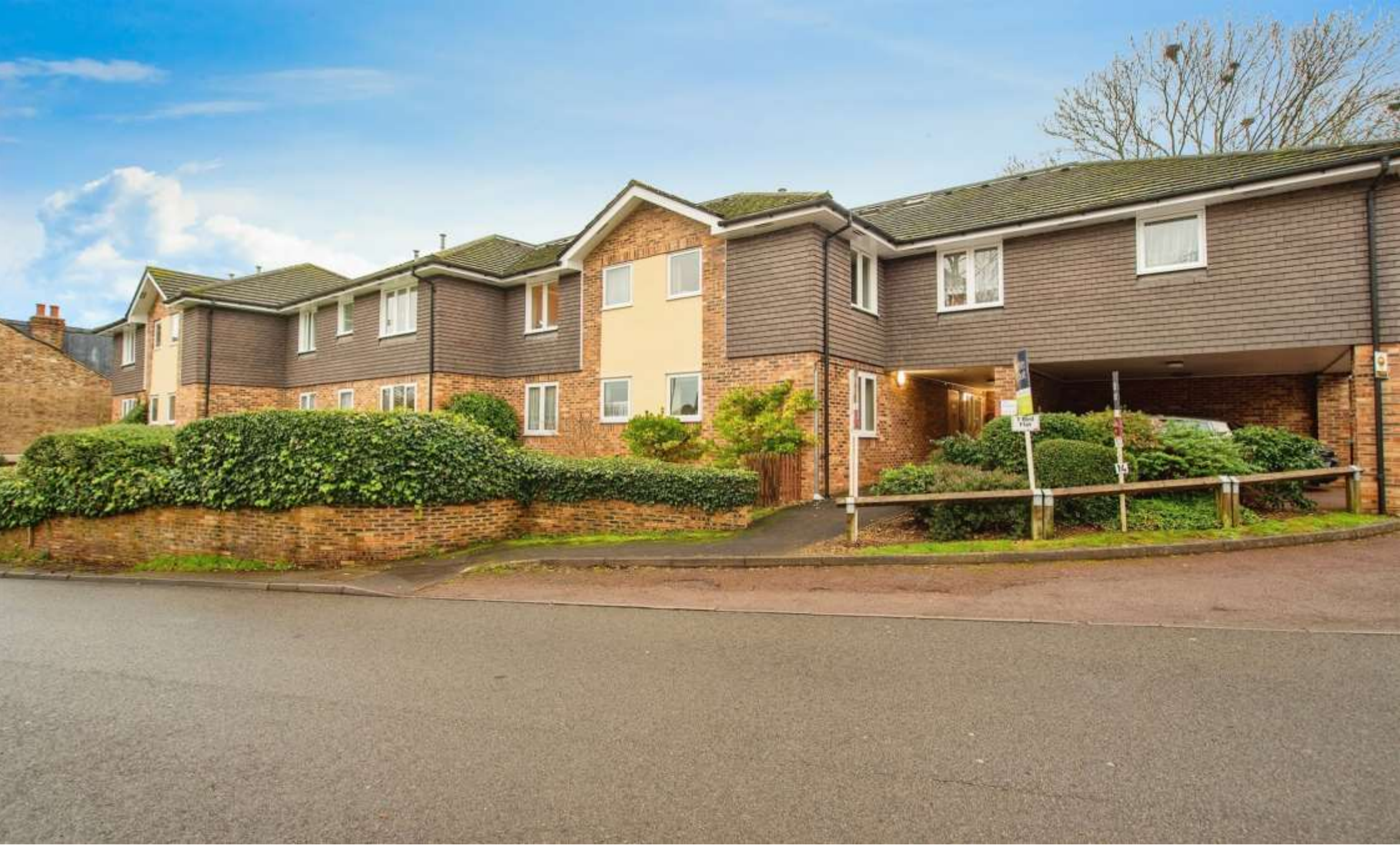
The Cloisters Church Lane, Kings Langley WD4 8JT
