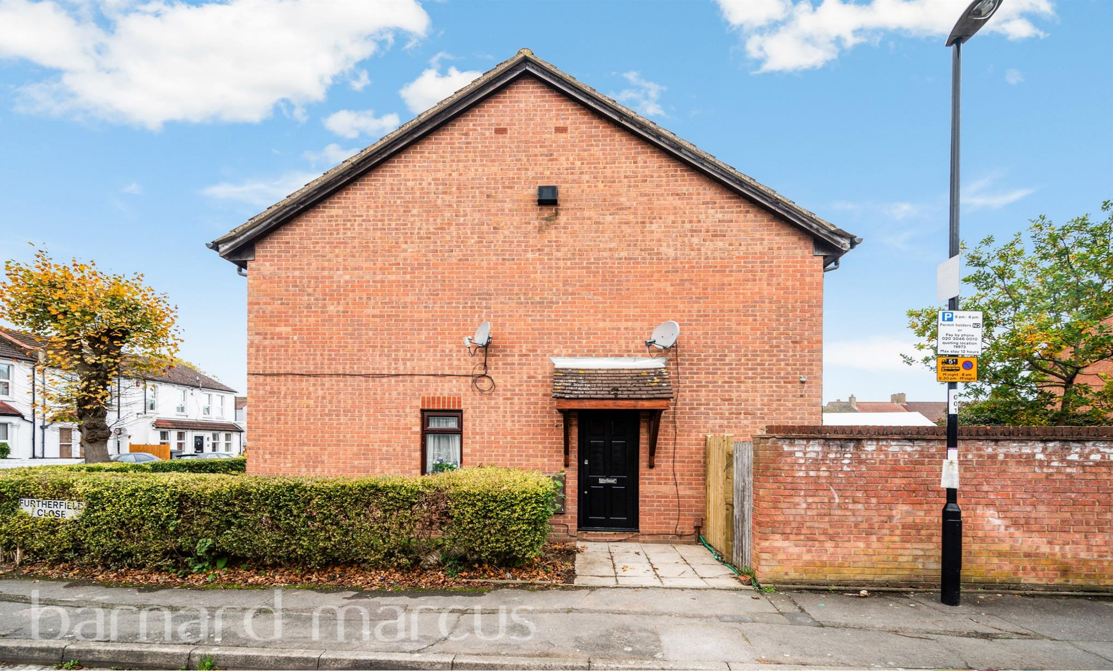
Furtherfield Close, Croydon CR0 3DZ
