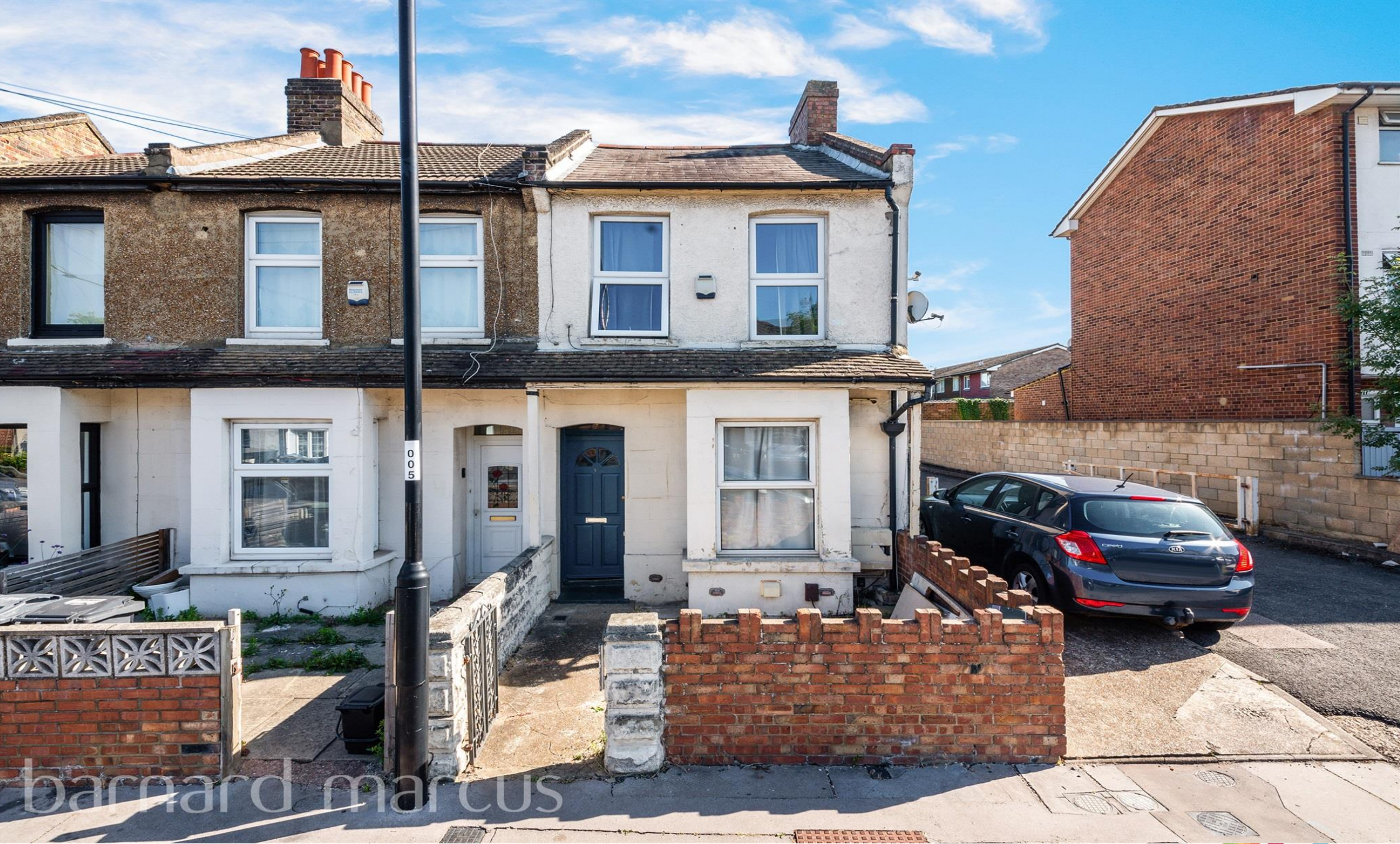
Osborne Road, Thornton Heath CR7 8PB
