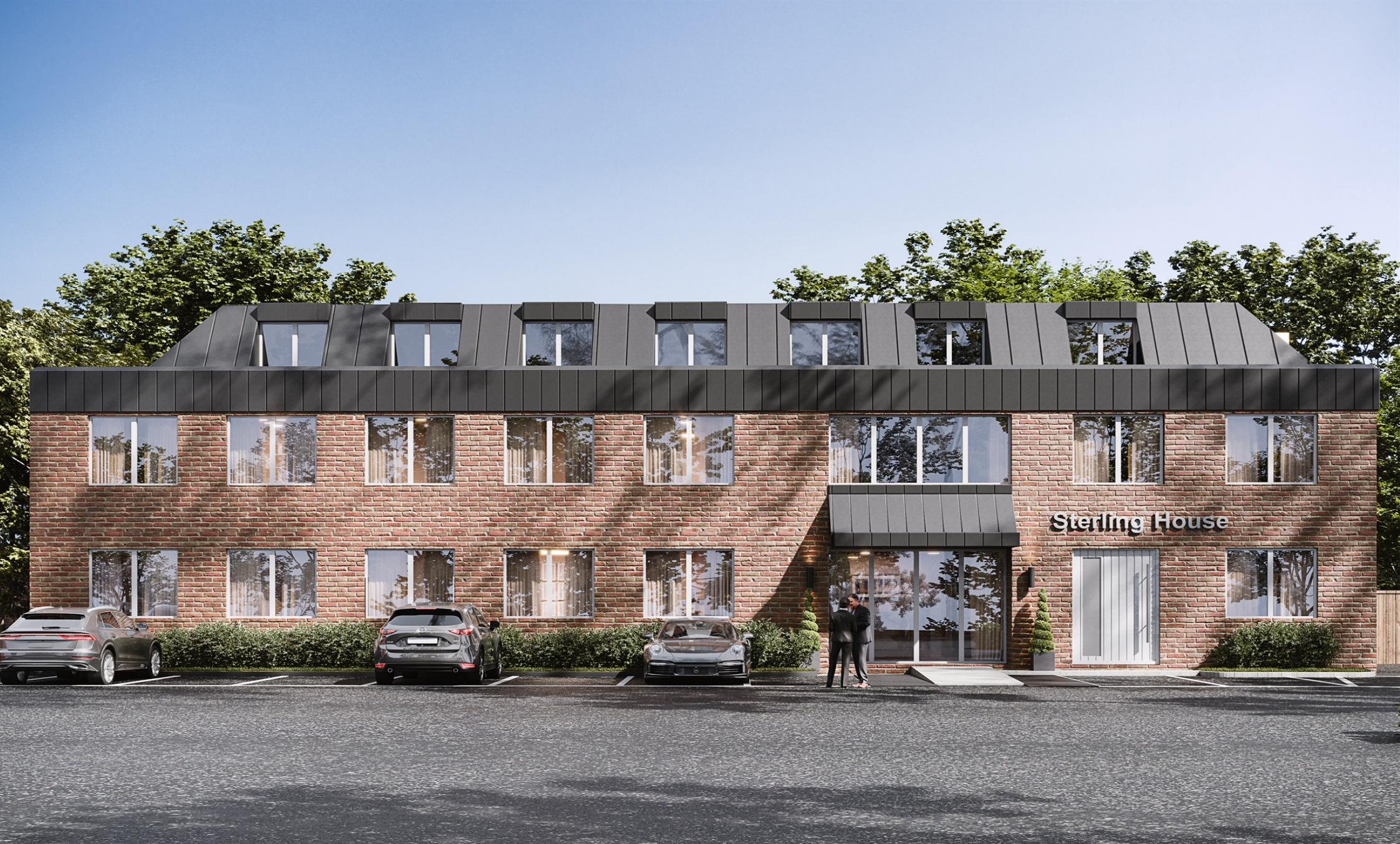
Sterling House Bolters Lane, Banstead SM7 2AR
