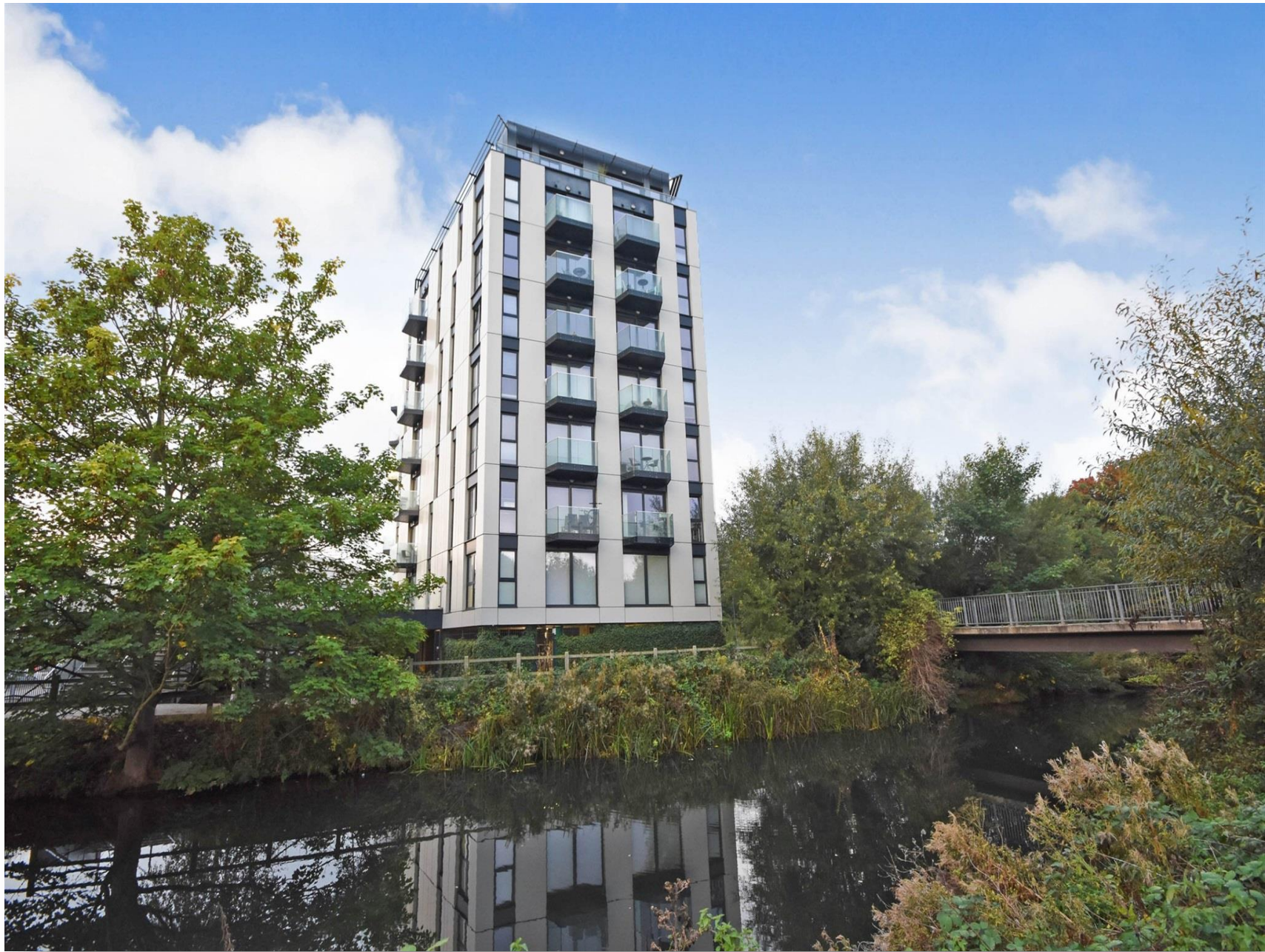
Shire Gate, City Centre Chelmsford CM2 0FQ
