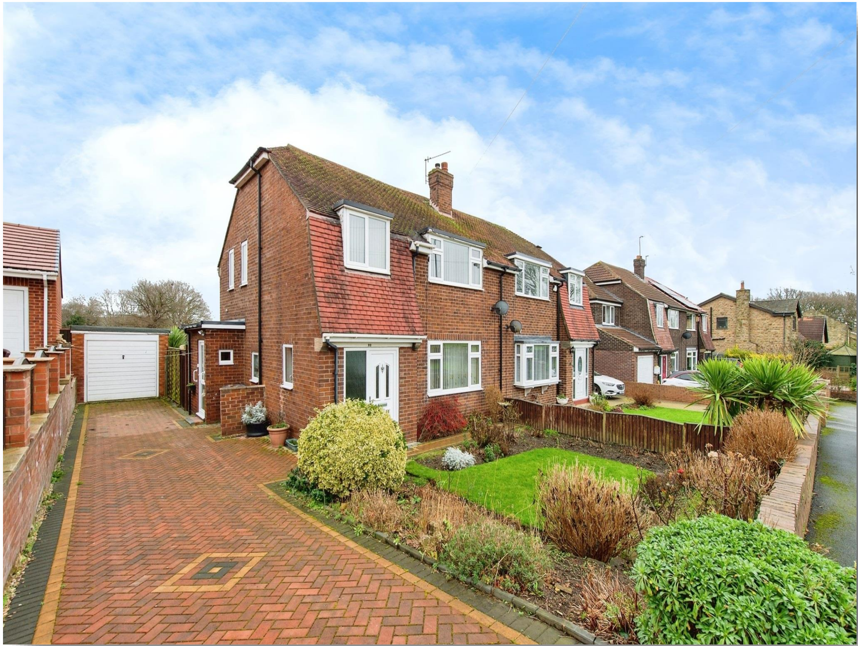
Leeds Road, Methley Leeds LS26 9EQ
