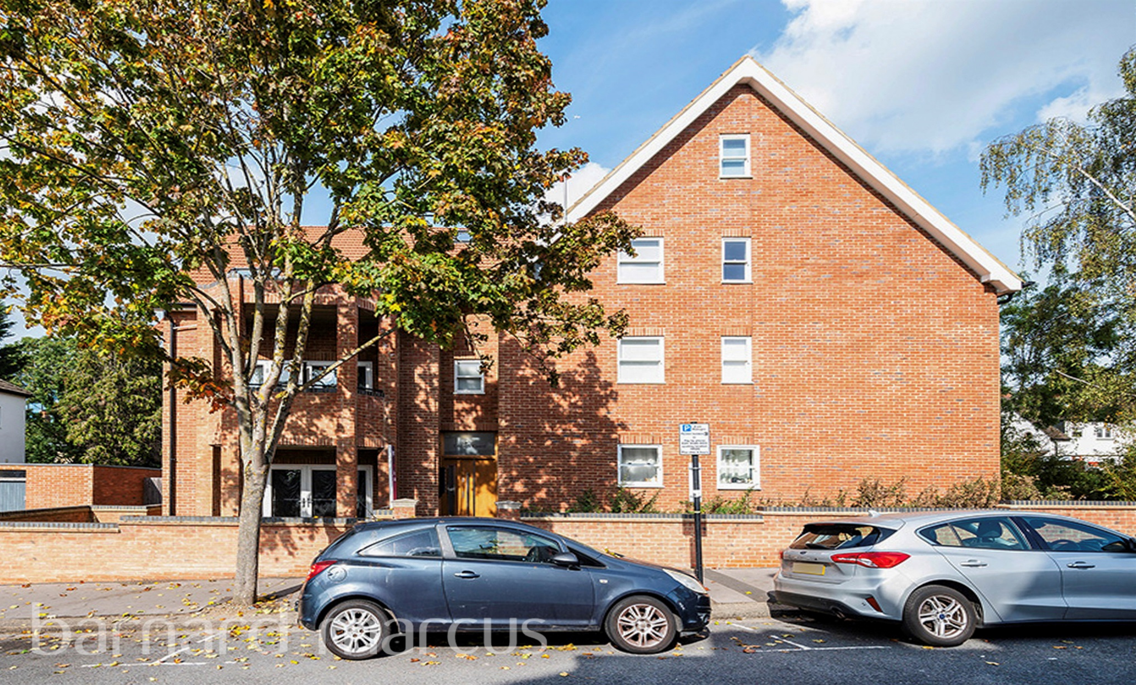
Emlagh Court Beech House Road, Croydon CR0 1JQ
