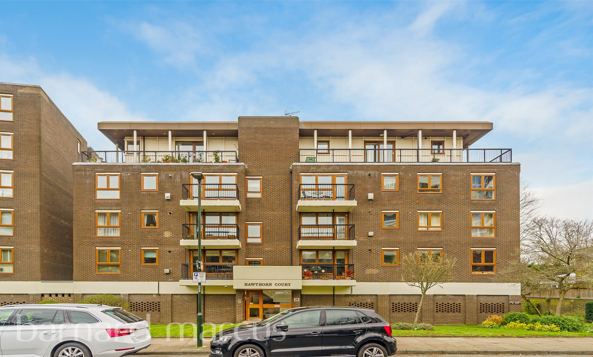
Hawthorn Court, Warwick Drive, London, SW15 6LF
