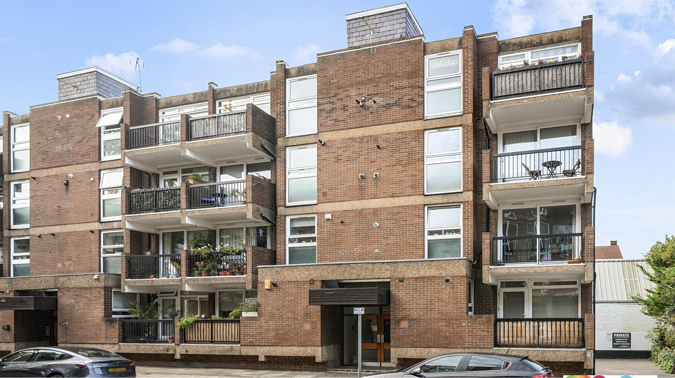
Sheridan House Wincott Street, London SE11
