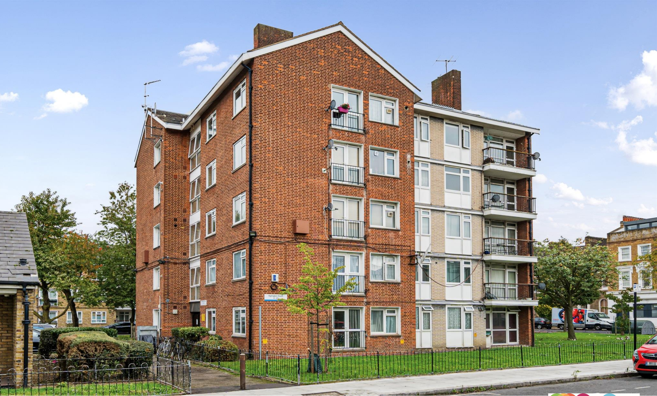
Eglington Court Lorrimore Road, London SE17
