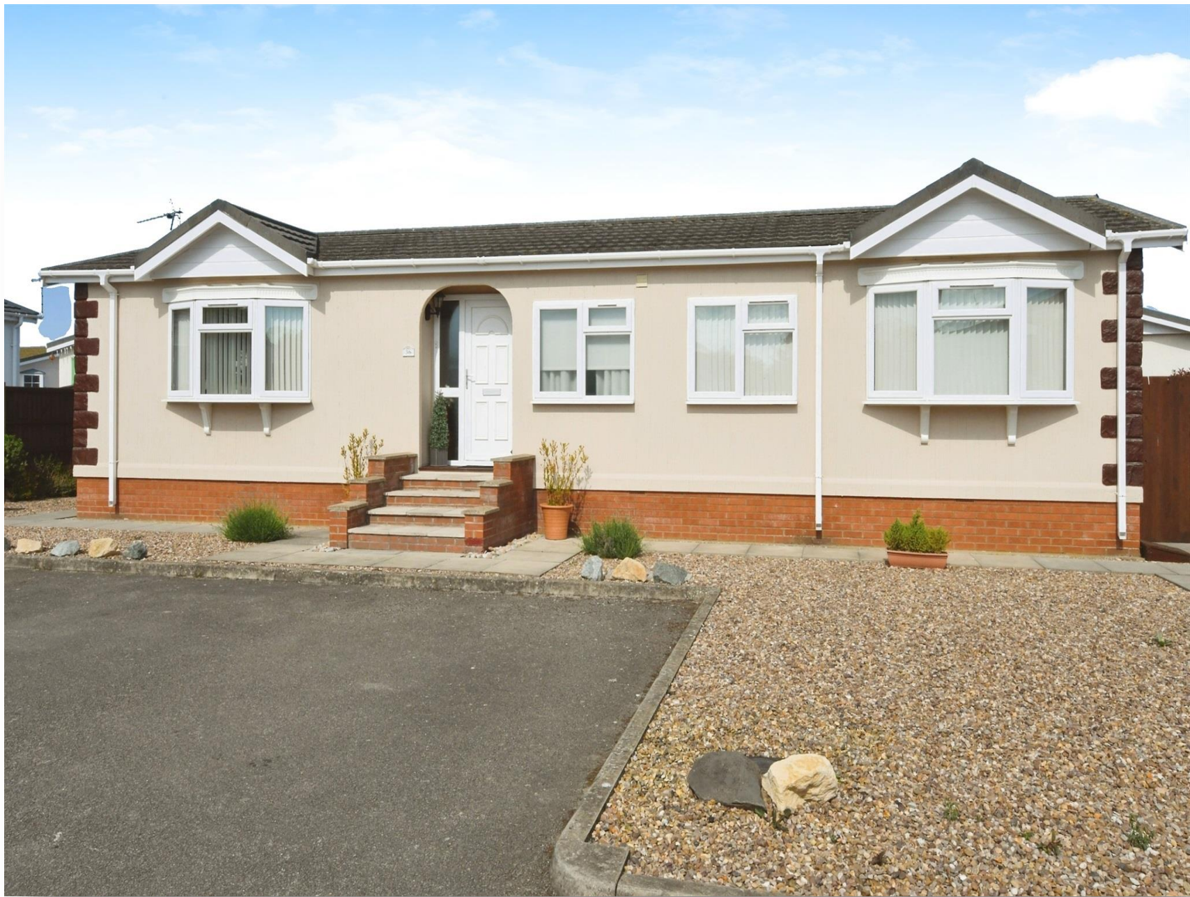
Hall Hills Park Tattershall Road, Boston PE21 9SG
