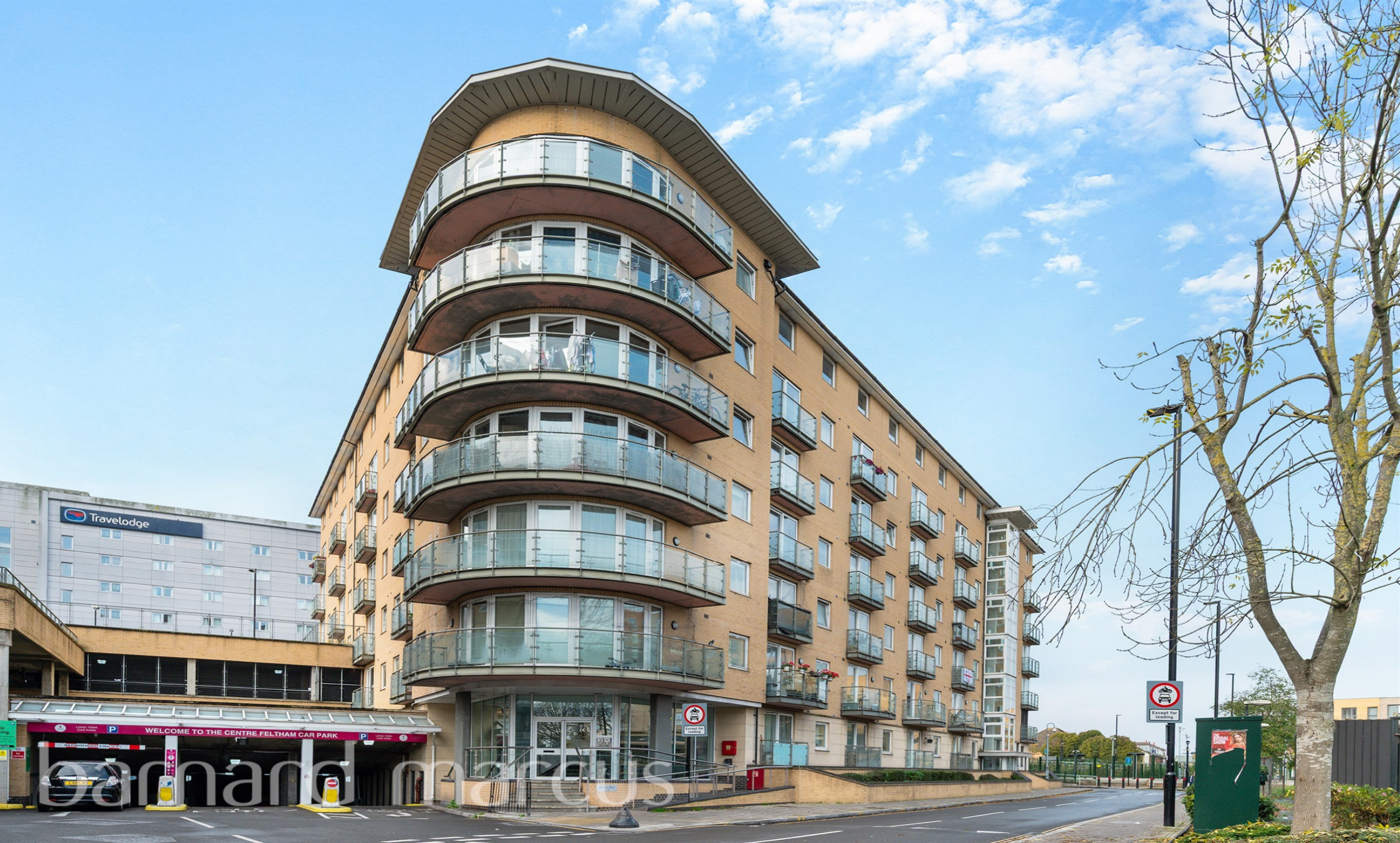
Bergenia House Bedfont Lane, Feltham TW13 4GE
