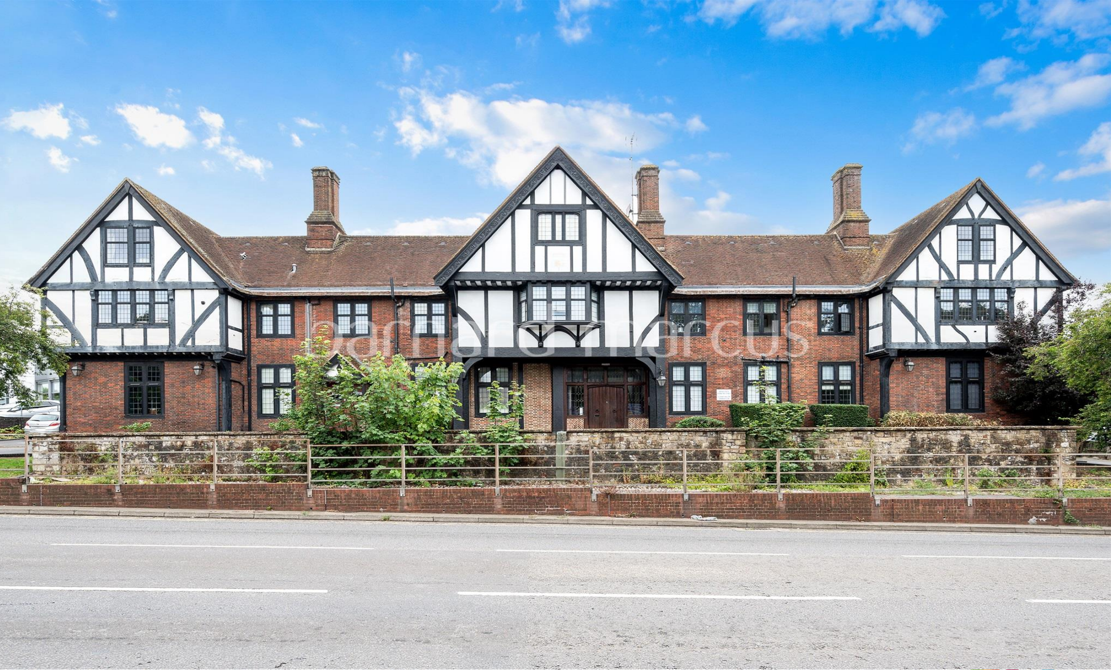
The Driftbridge Reigate Road, Epsom KT17 3JZ
