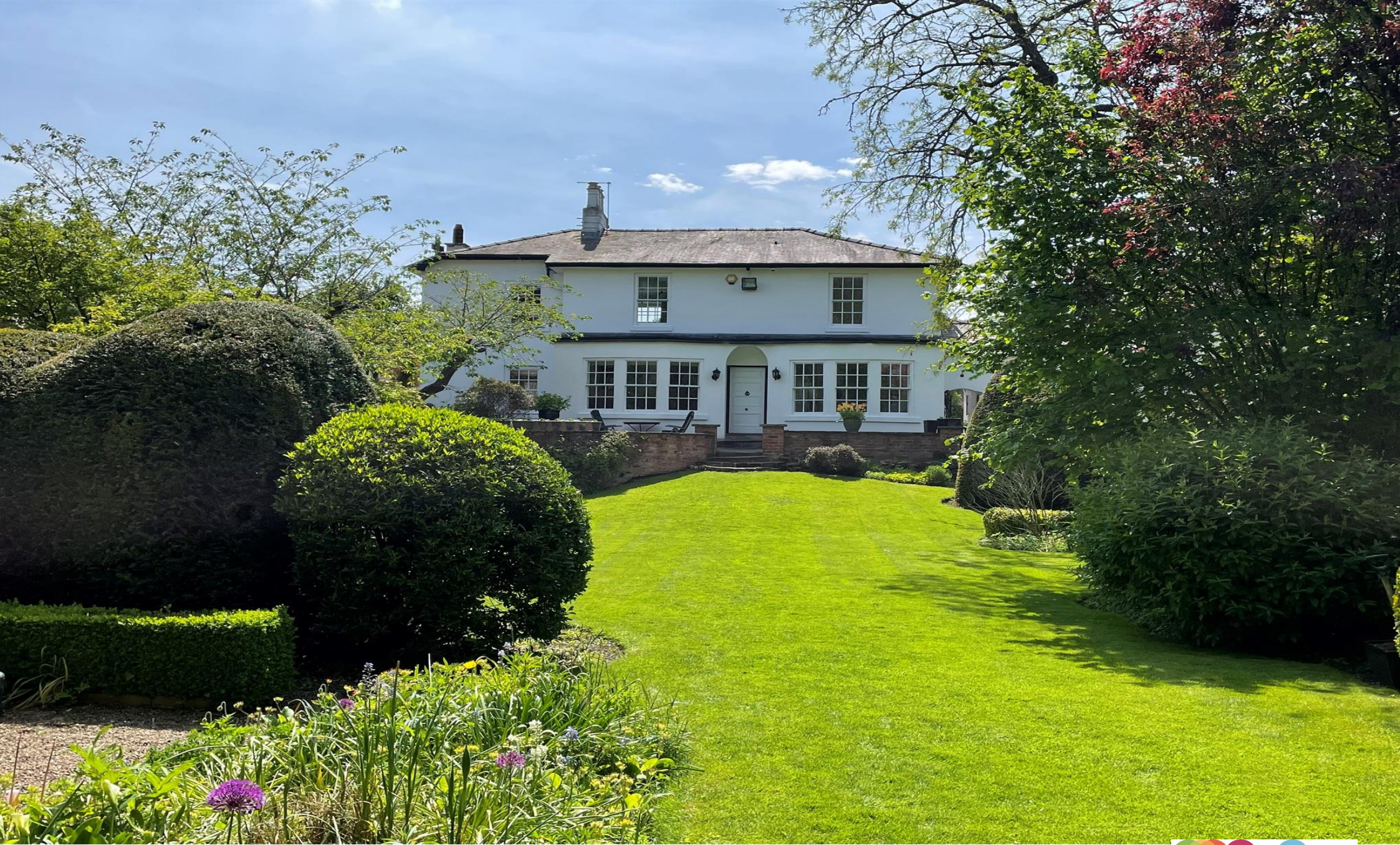
Brook House, Lindrick Road, Tickhill, Doncaster DN11 9RD
