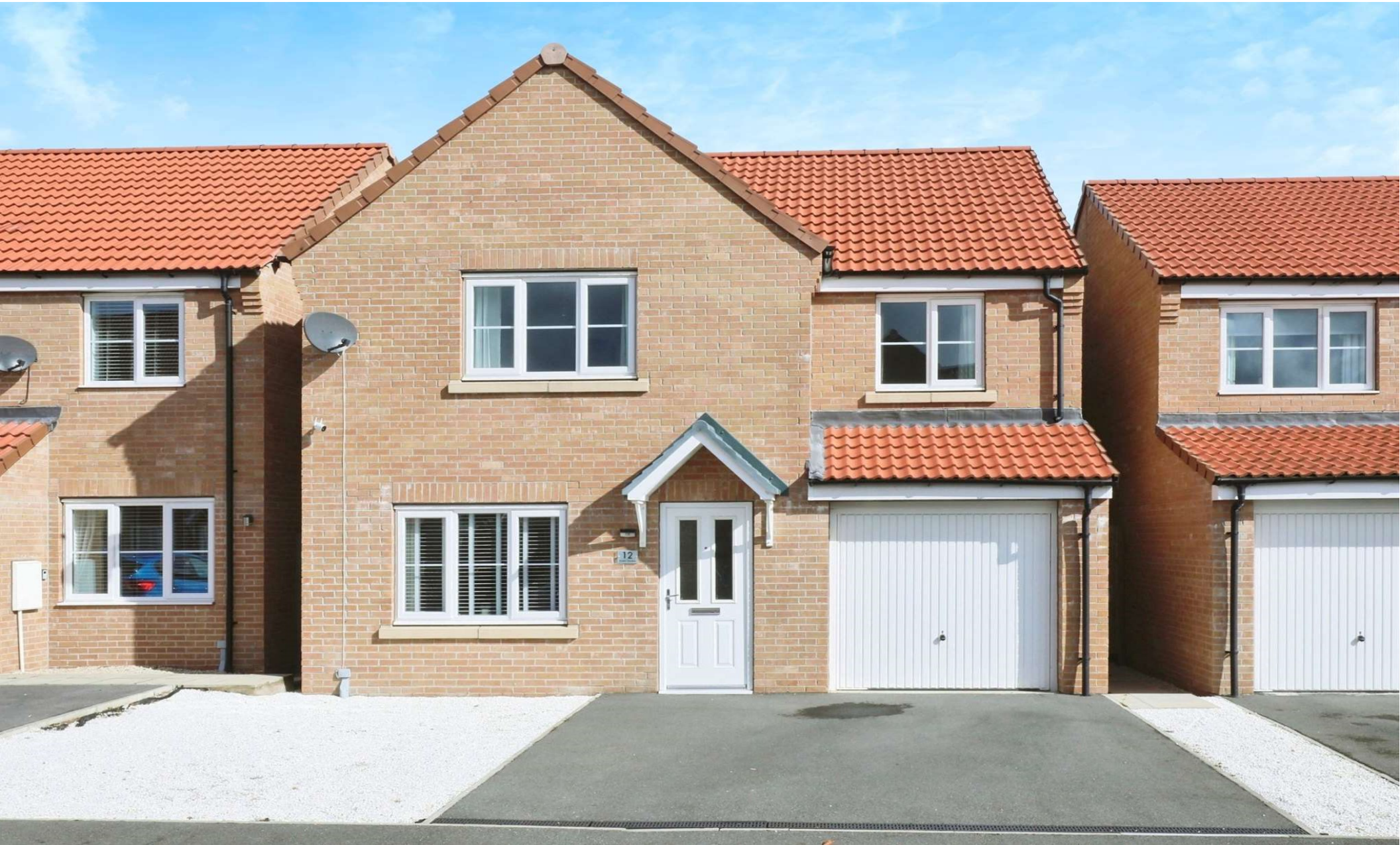
Avalon Gardens, Harworth Doncaster DN11 8FD
