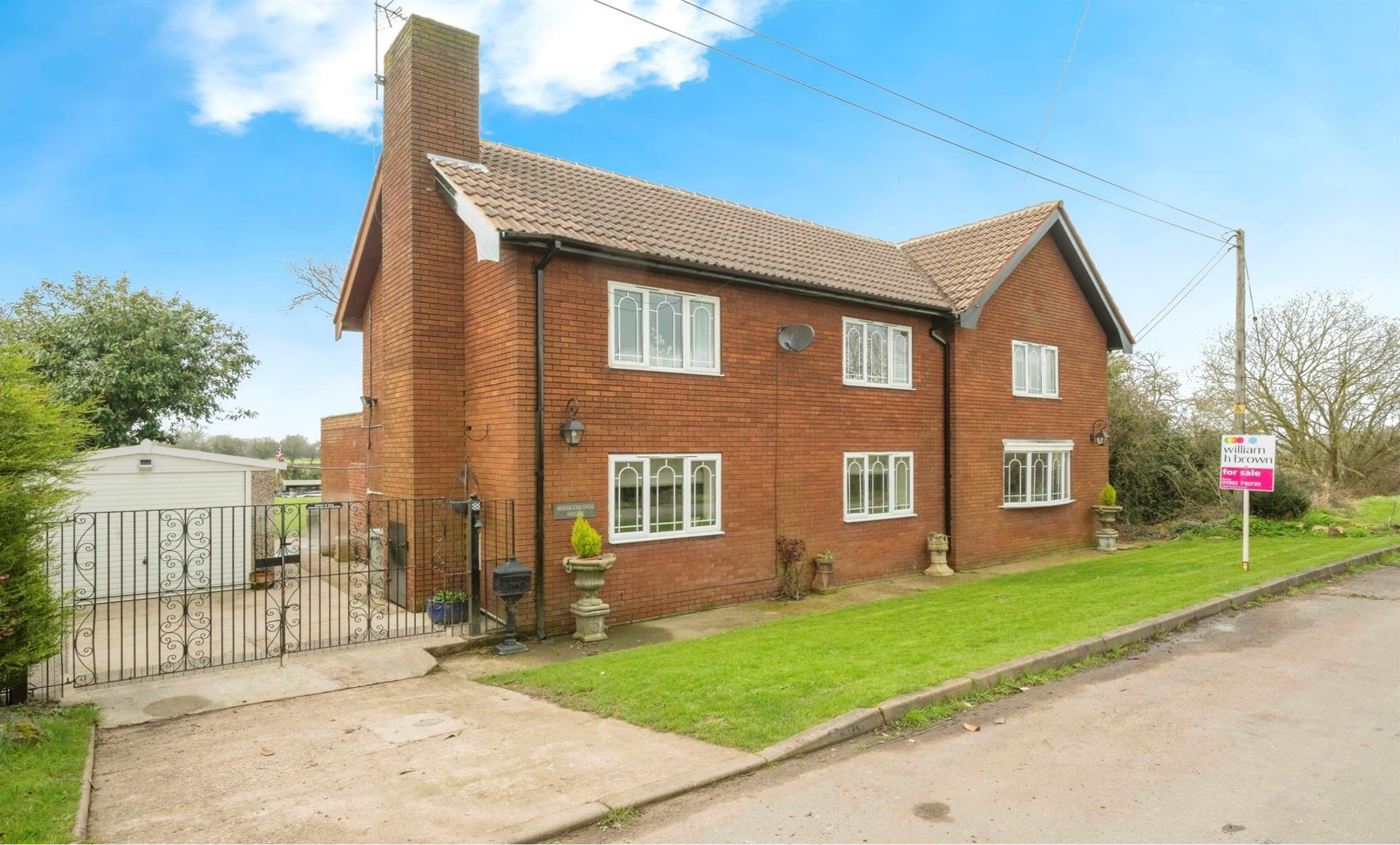
Middlebridge House Middlebridge Road, Gringley-On-The-Hill Doncaster DN10 4SE
