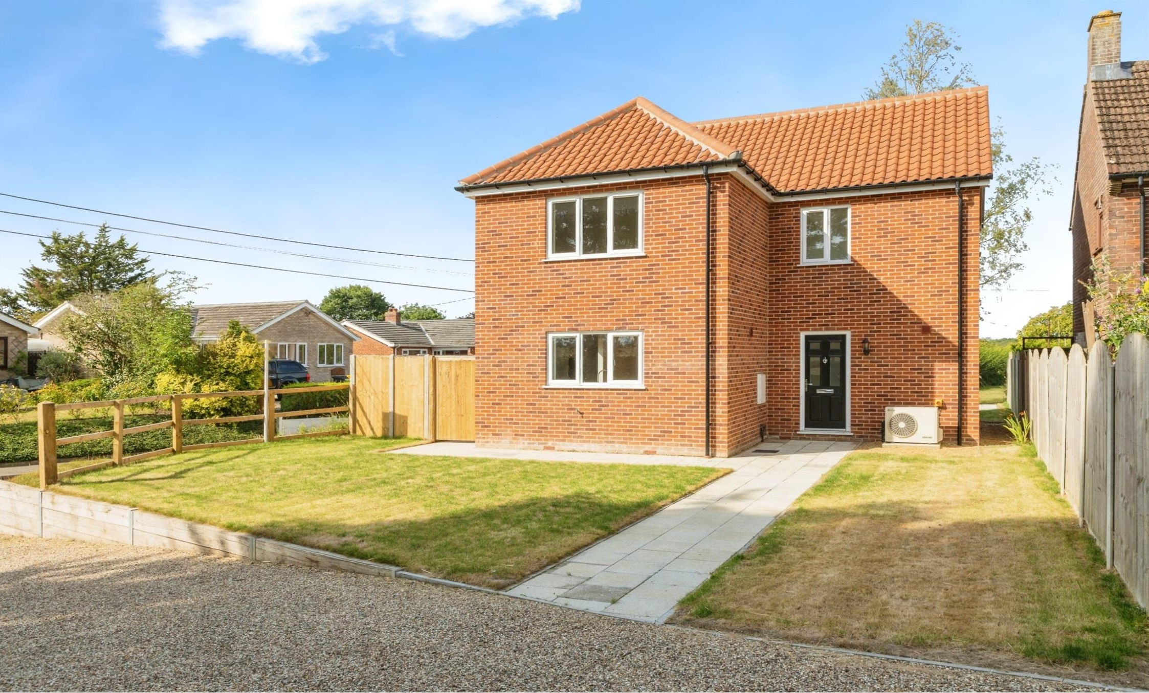
Winfarthing Road, Banham Norwich NR16 2HA
