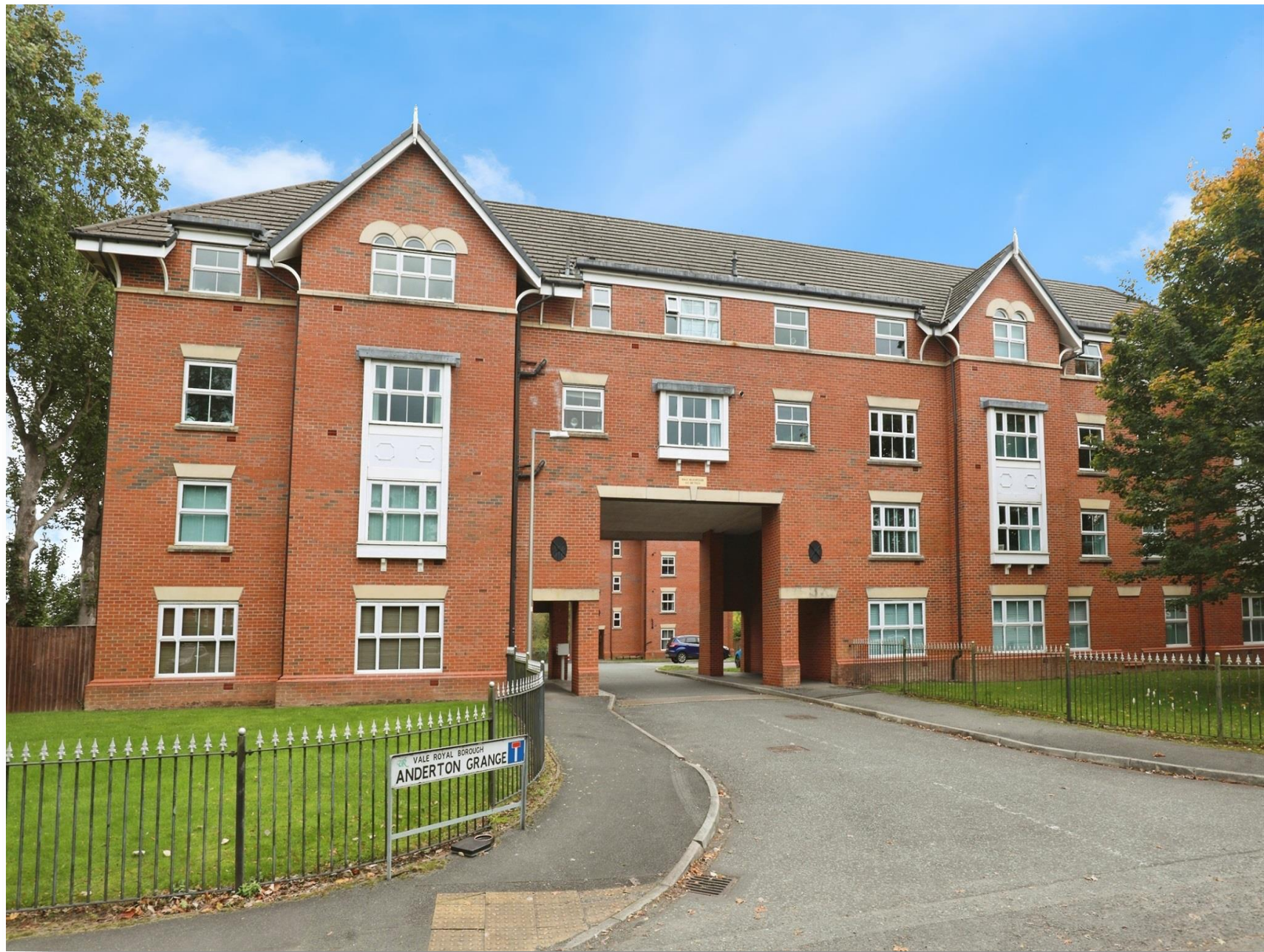
Anderton Grange Hollands Road, Northwich CW9 8PY
