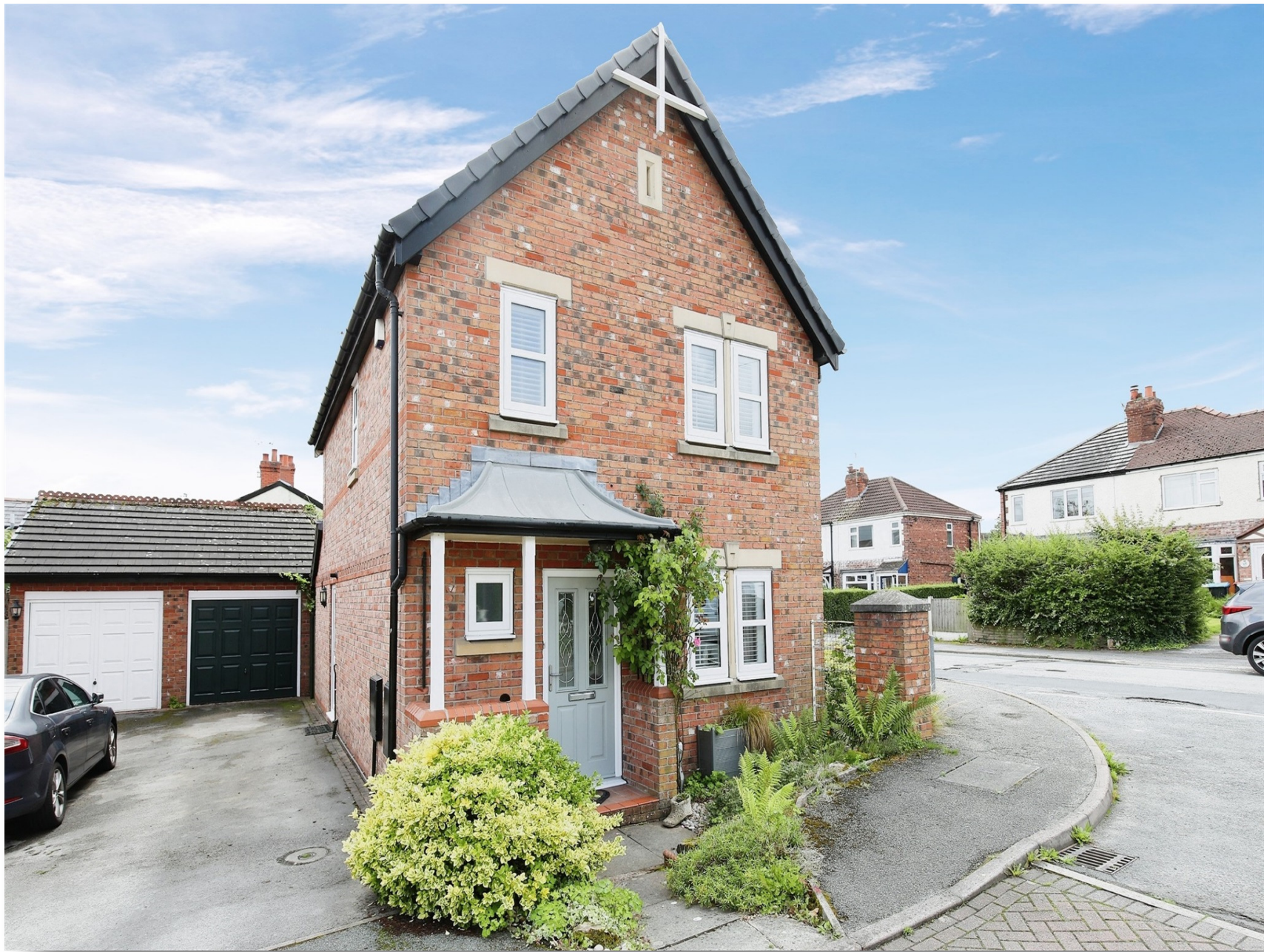
Ashley Grange, Davenham Northwich CW9 8HJ
