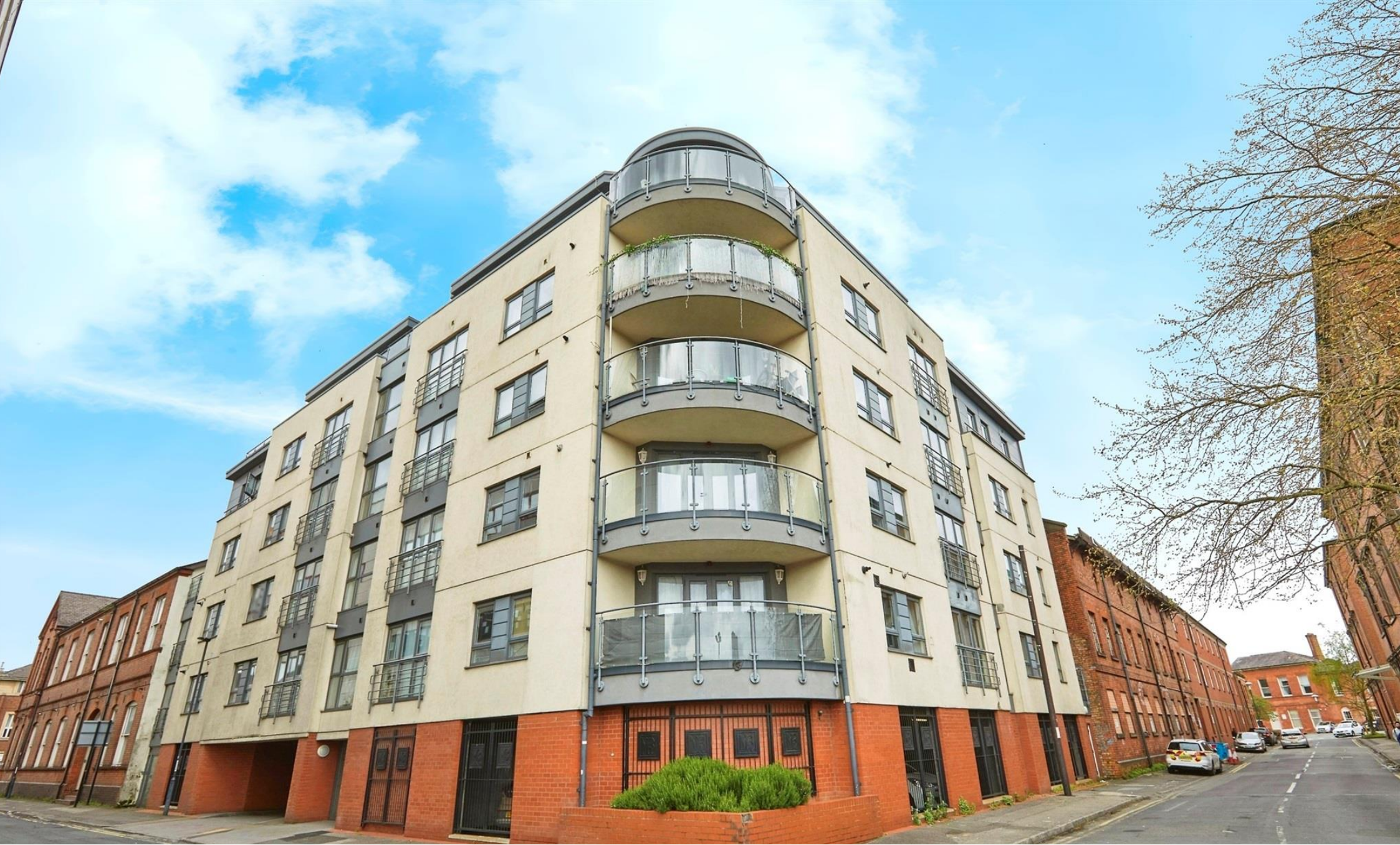
Rutland House Carrington Street, DERBY DE1 2NH
