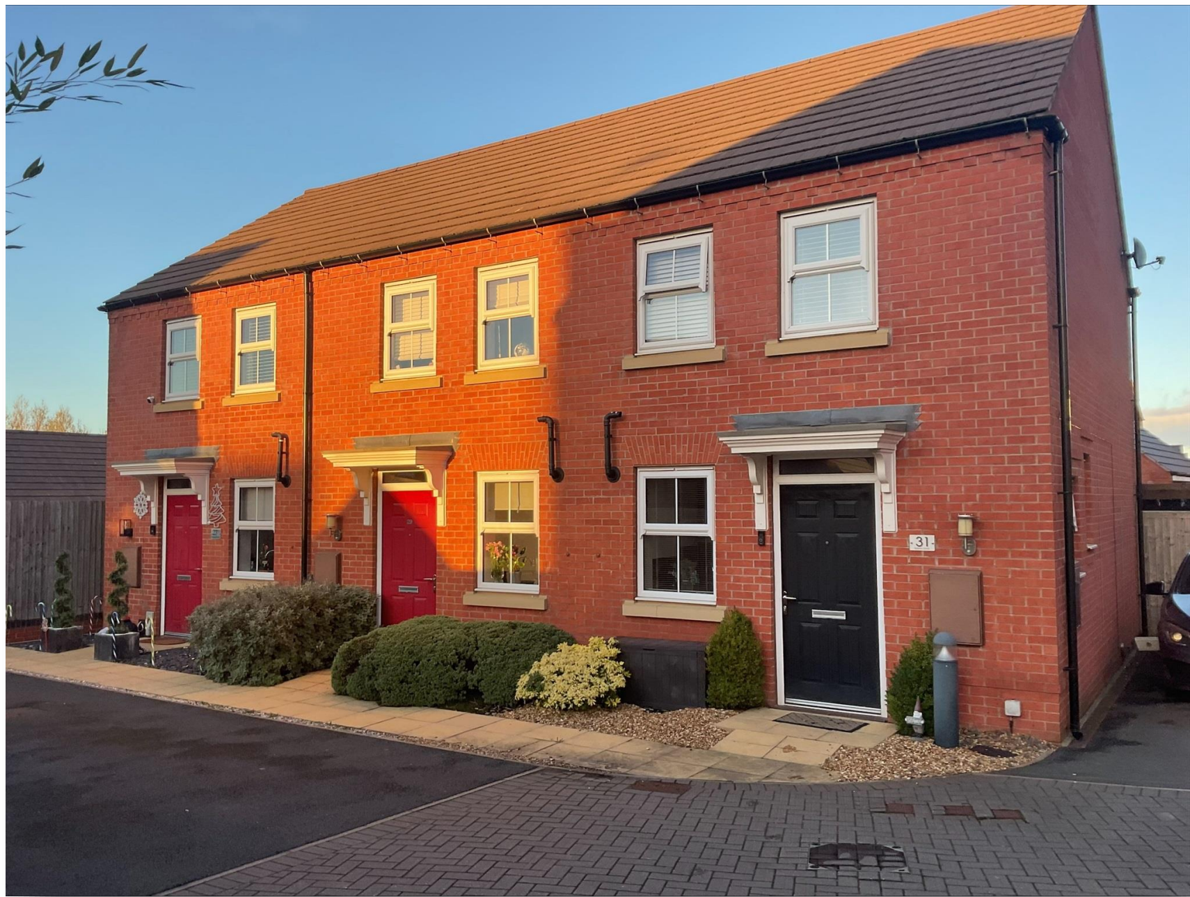
Barton Drive, Ashbourne DE6 1TN
