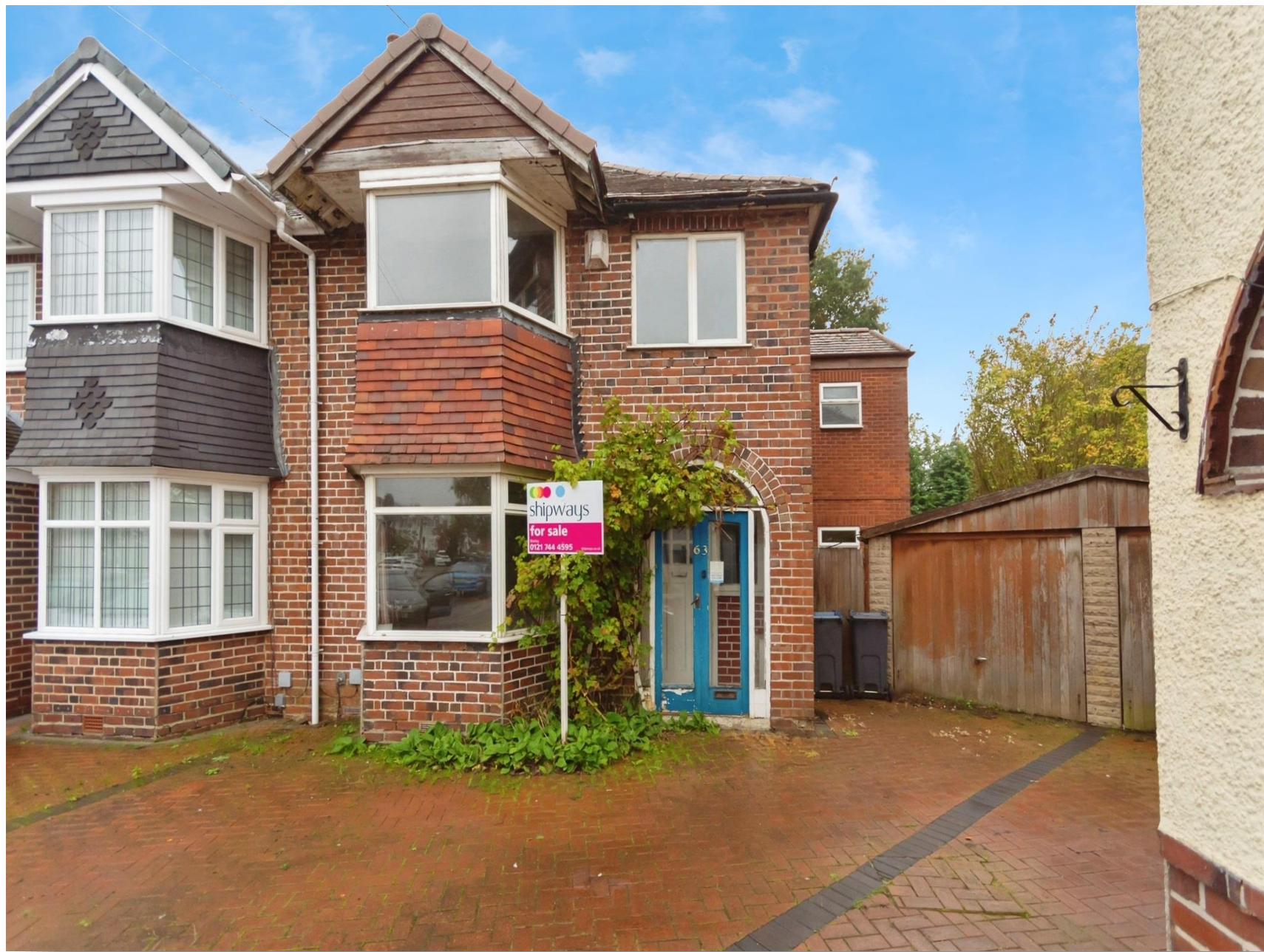
Hilton Avenue, Birmingham B28 0PE
