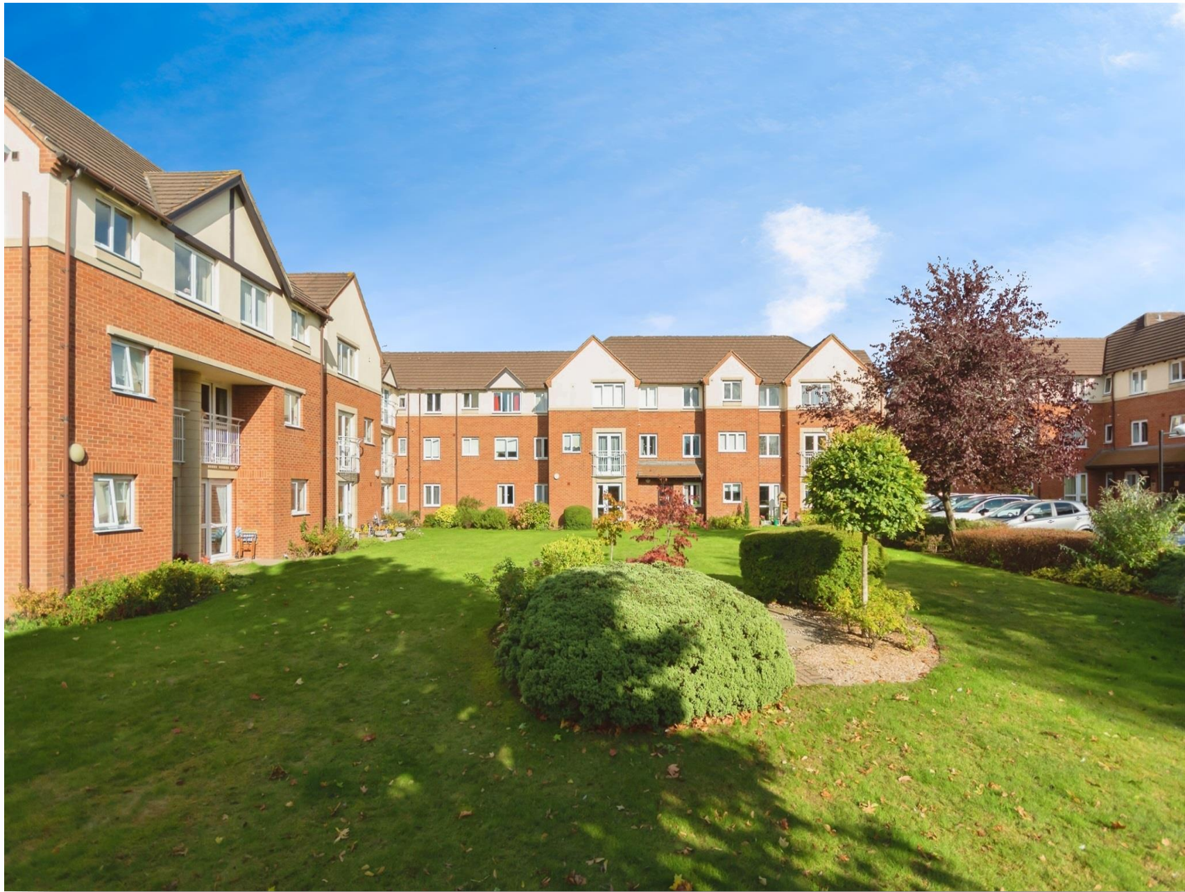
Rivendell Court Stratford Road, Hall Green Birmingham B28 8AT
