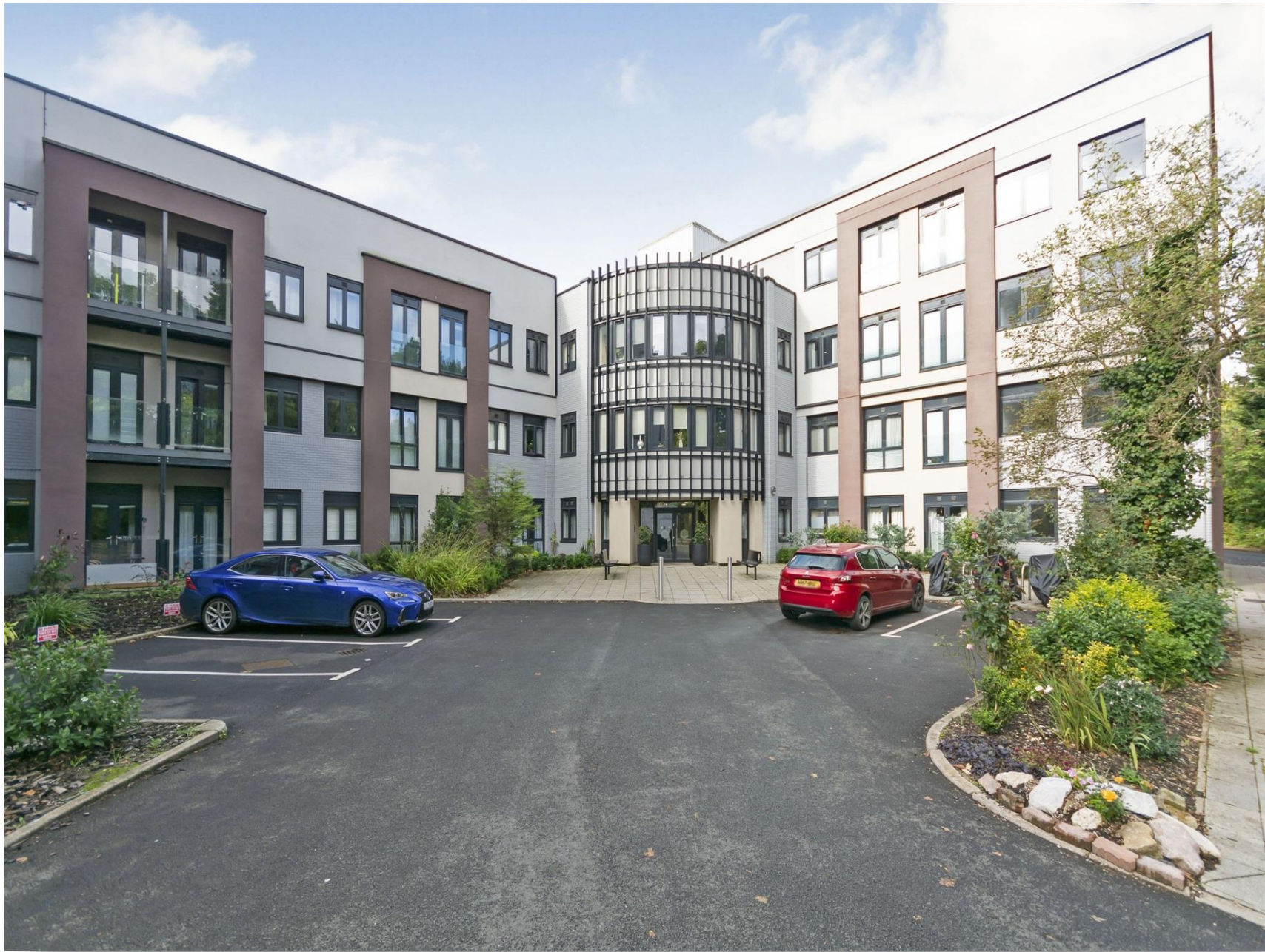
Broadoaks Streetsbrook Road, Solihull B91 1QY
