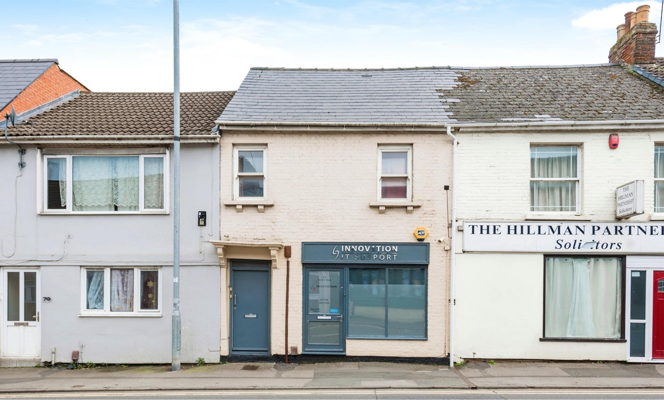
Victoria Road, Swindon SN1 3BB
