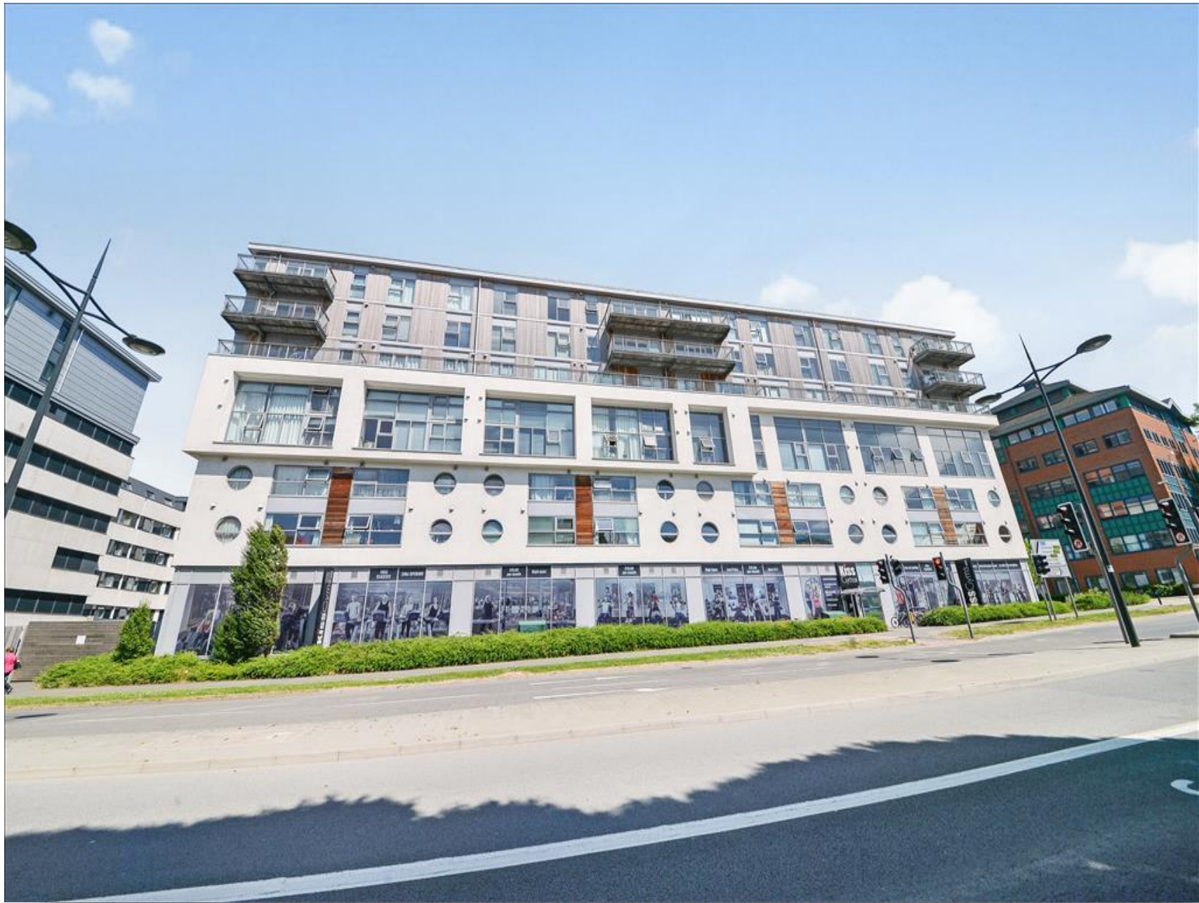
Paramount Beckhampton Street, Swindon SN1 2SB
