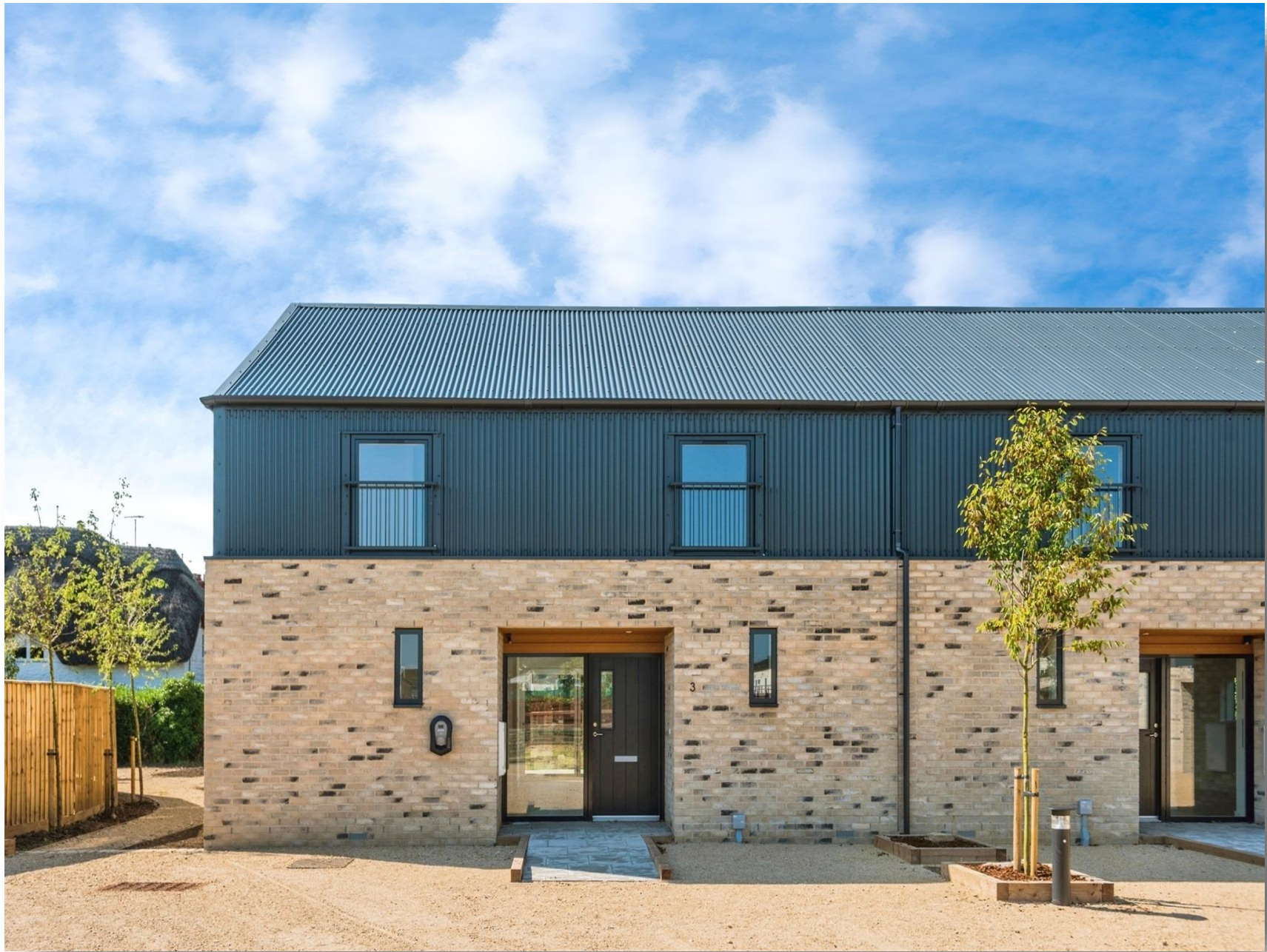
The Limes Green Road, Stratton St Margaret, Swindon SN2 7JE
