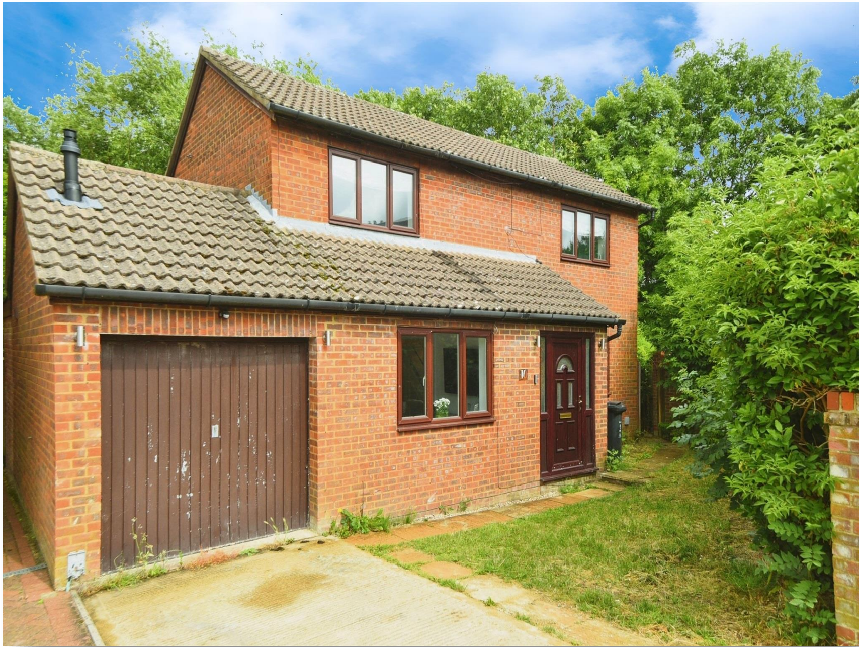
Sandpiper Bridge, Swindon SN3 5DY
