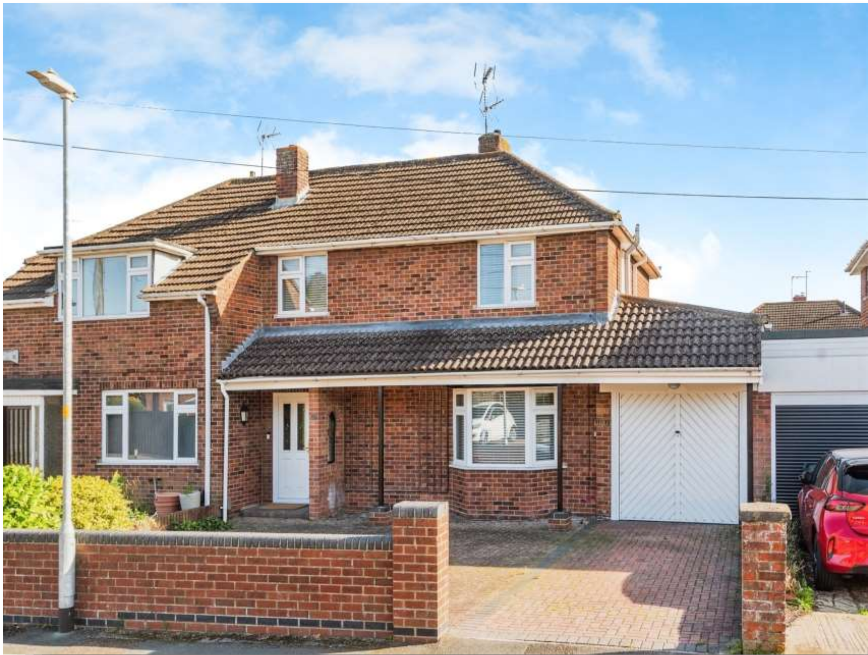
Burns Way, Swindon SN2 7LP
