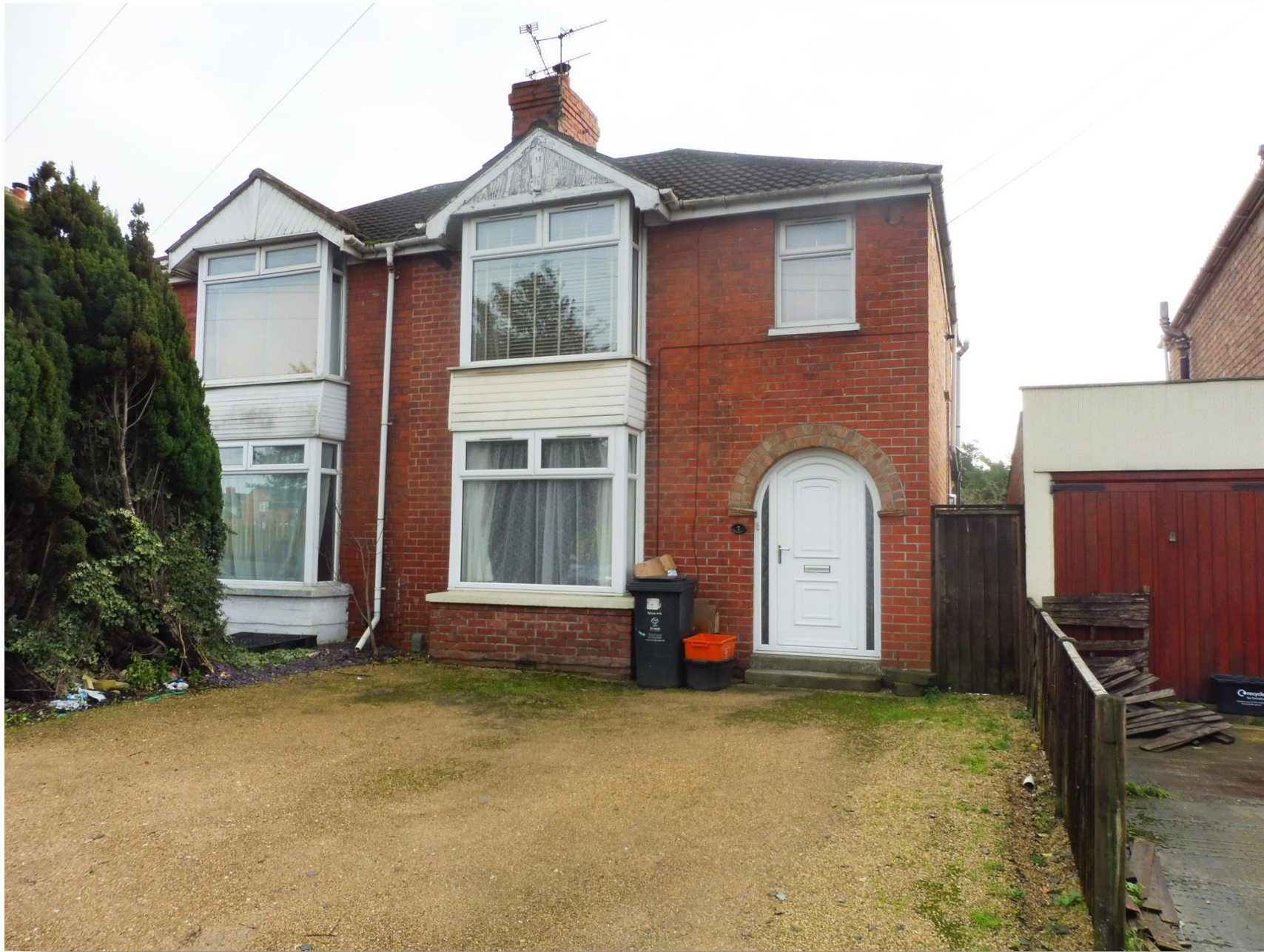
Bridge End Road, SWINDON SN3 4PD
