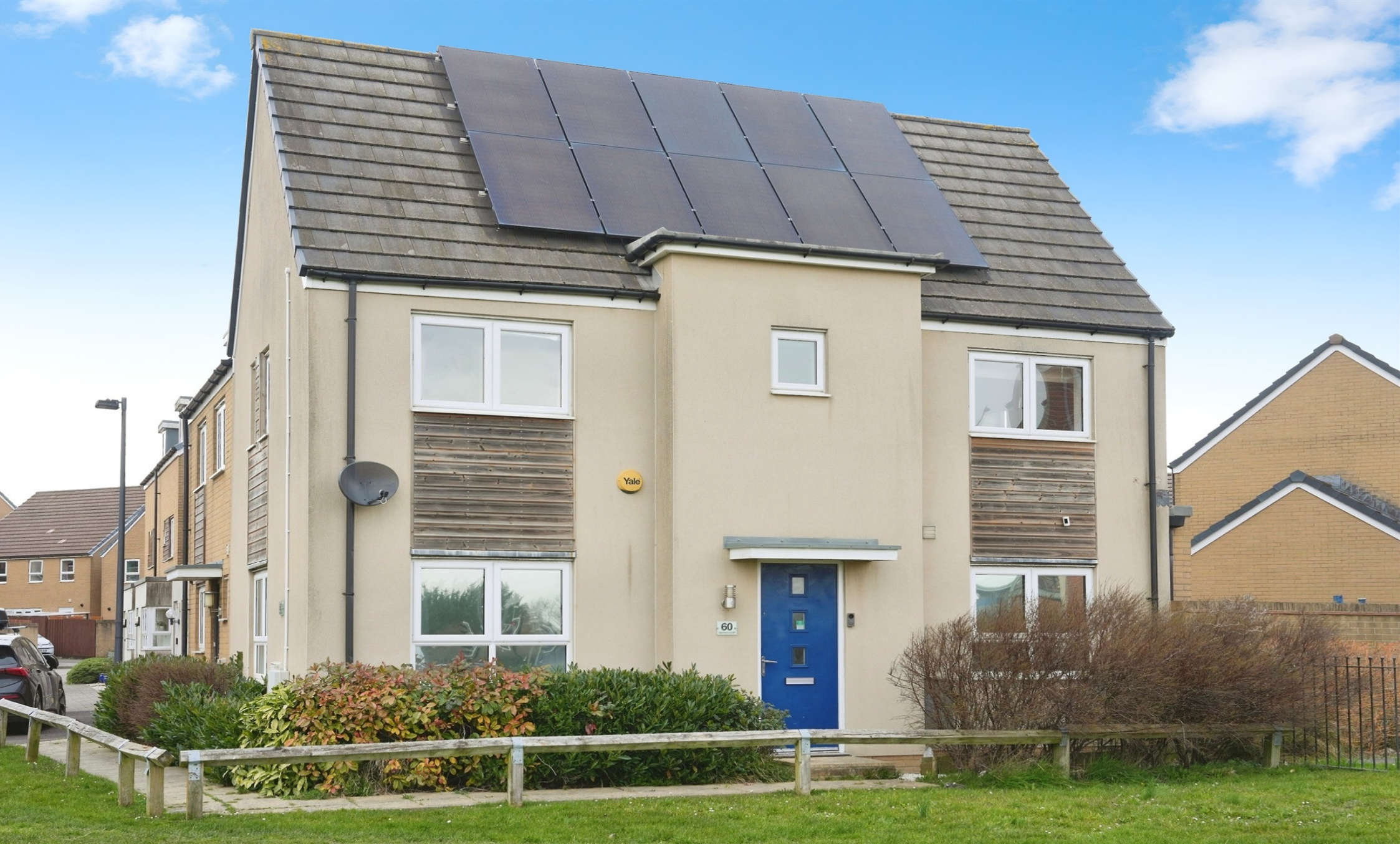
Skidders Croft, Patchway Bristol BS34 5AX
