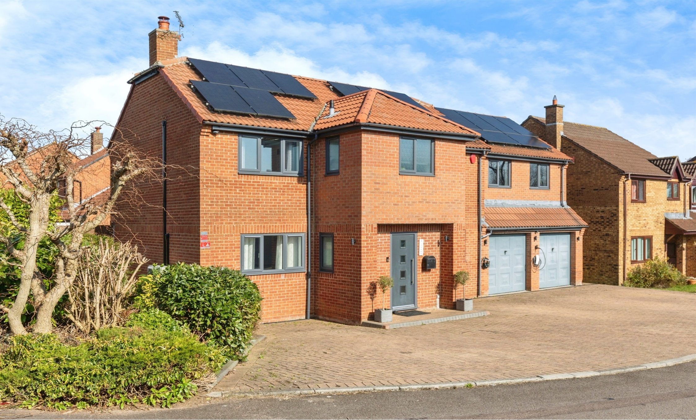
Grange Close, Bradley Stoke BRISTOL BS32 0AH
