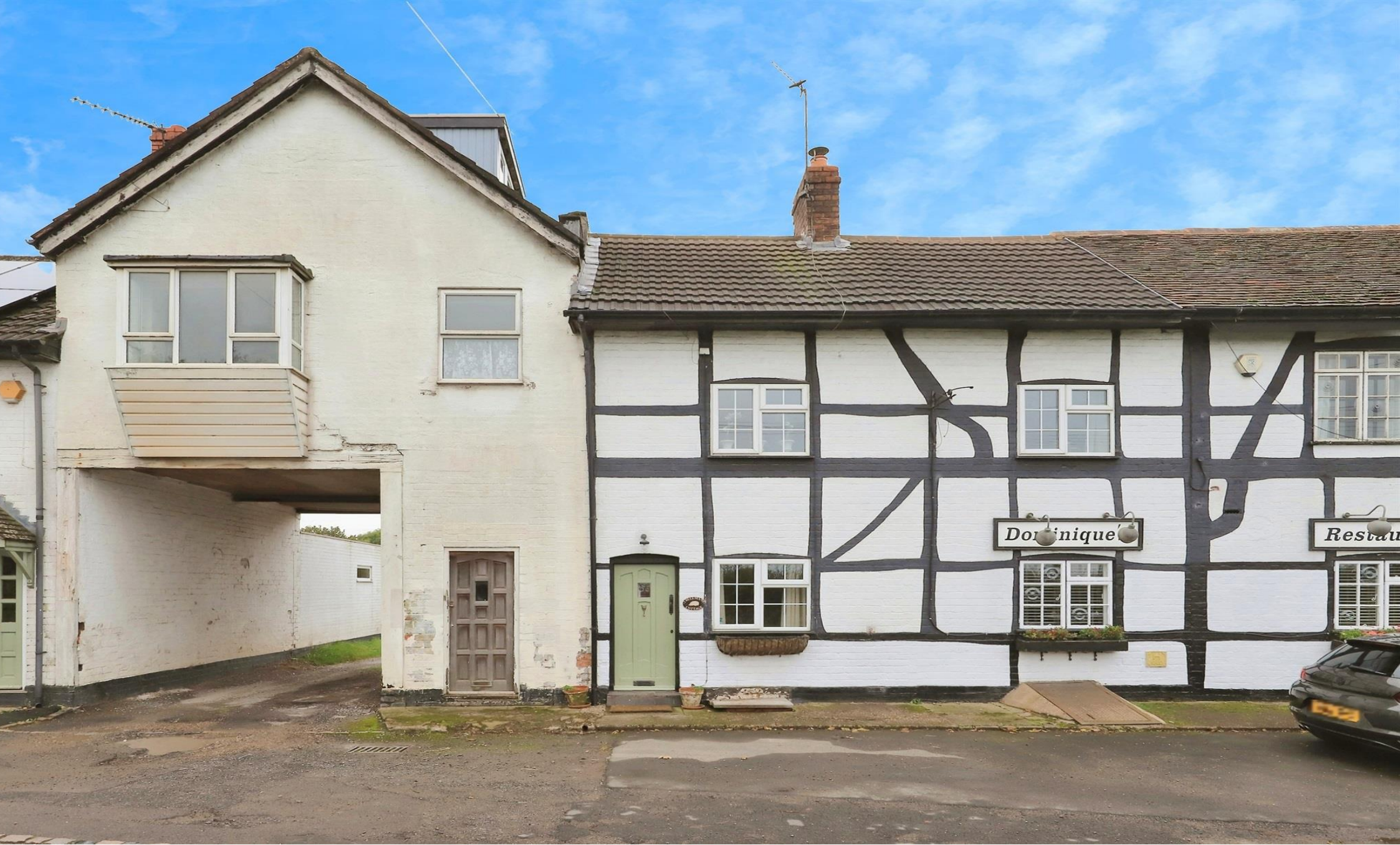
Bellmans Cottages, Shatterford Bewdley DY12 1RN
