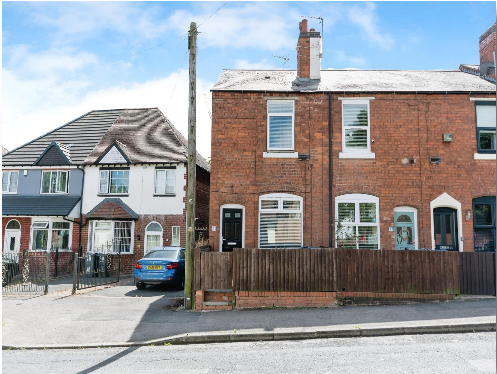
Jiggins Lane, Birmingham, B32 3LA
