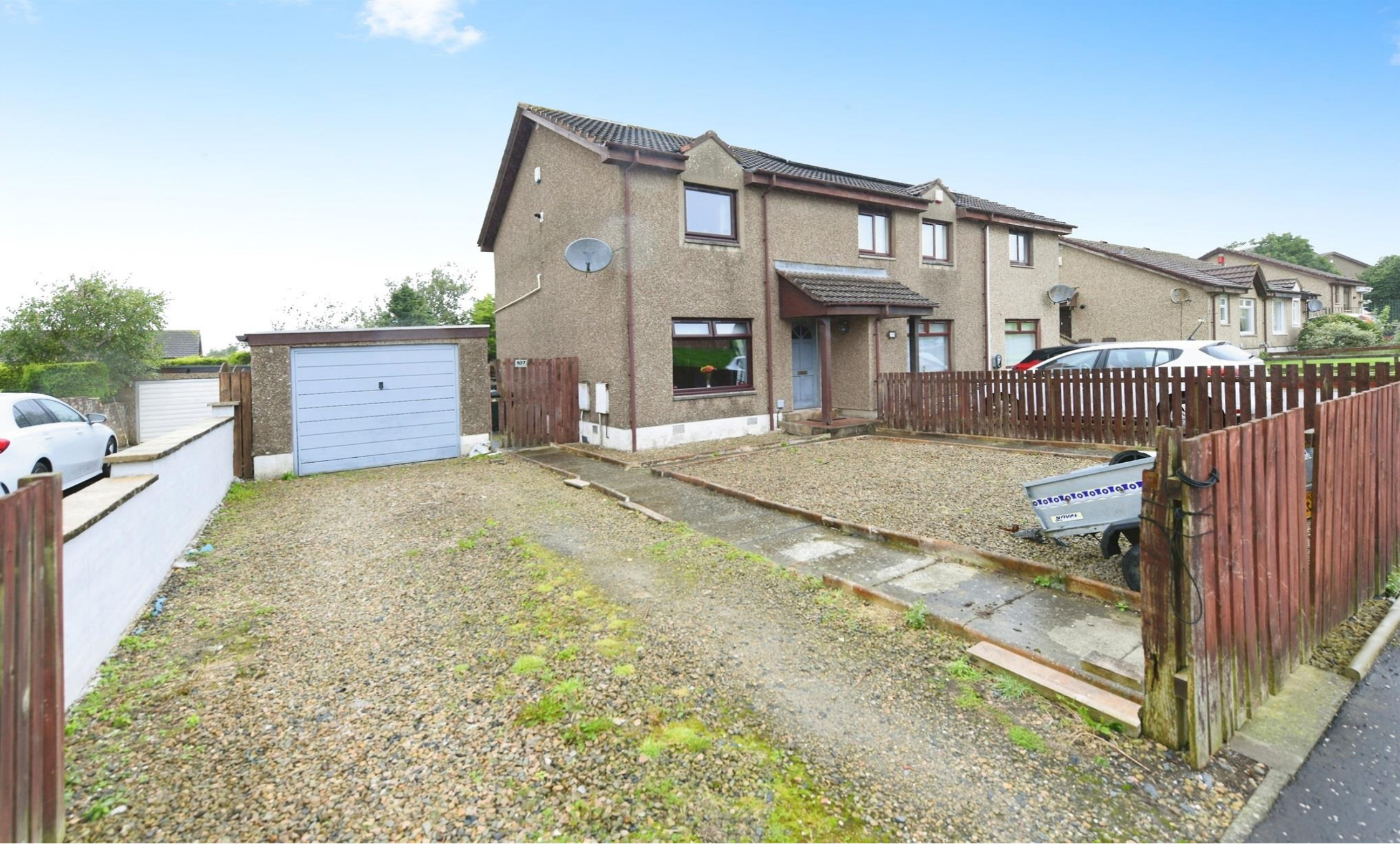
Bridgehousehill Road, Kilmarnock KA1 4QB
