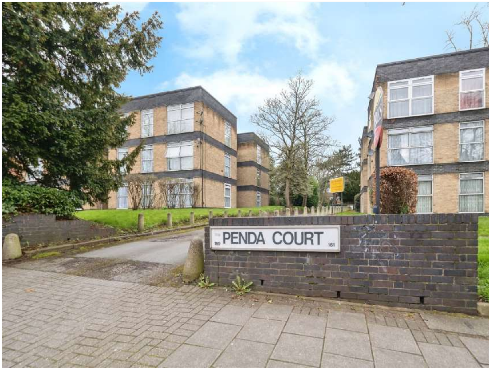
Penda Court Hamstead Road, Handsworth Birmingham B20 2RL
