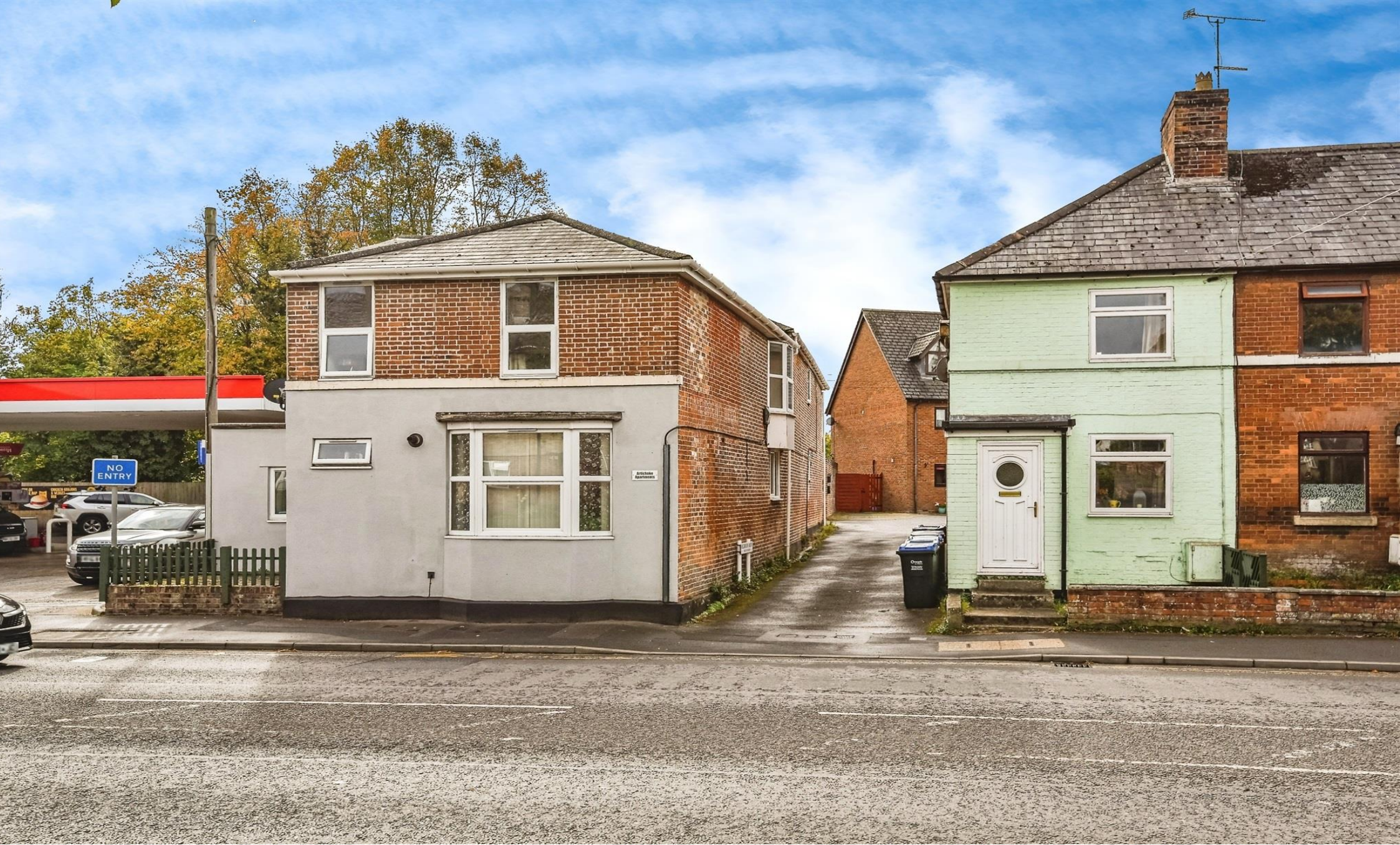
The Old Artichoke Apartments, The Nursery, Devizes SN10 2AA
